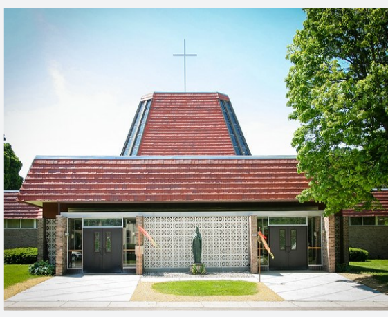
EAST SITE 2322 S. 106th Street
