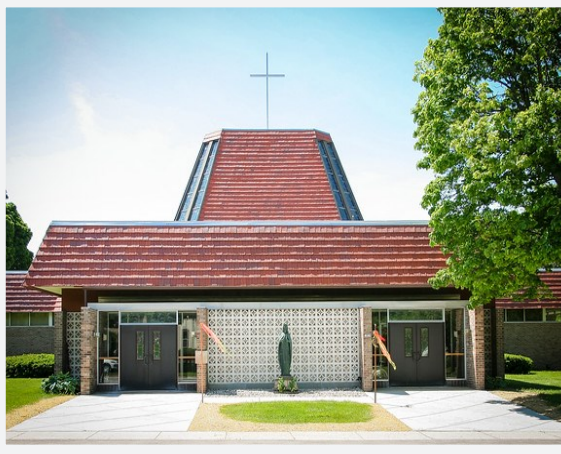
EAST SITE 2322 S. 106th Street
