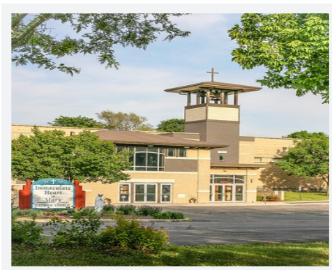
116TH STREET SITE 1212 S. 117th Street
