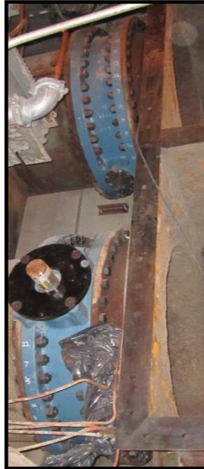
In 2014 & 2015 FreeState Flow Solutions supplied eight 48" and eight 54" Condenser Isolation valves to a power generation facility in the Midwest. The scope of work included reverse engineering custom mono-flange valves. These valves replaced the original valves that had been a costly maintenance problem at the facility for many years.
