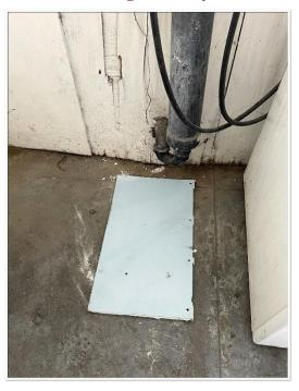
Large hole partially covered with metal plate is a possible trip hazard and a possibility of foot or feet falling into the exposed portion of hole. This is a safety concern. We advise repair/replacement as needed to ensure safety.
