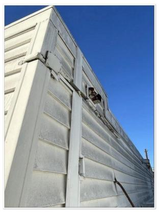
Running water dripping down from downspouts onto mailboxes; we advise making necessary corrections.
