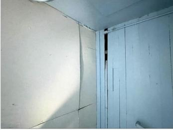
Holes, missing material and unknown opening in wall; unable to determine purpose; we advise making necessary corrections.
