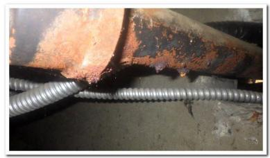
Corrosion noted at supply lines; no evidence of leakage at time of inspection.
