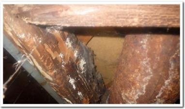
Excessive corrosion noted at drain lines at various areas; no leak at time of inspection; suggest consulting with specialist for further review prior to close of escrow.
