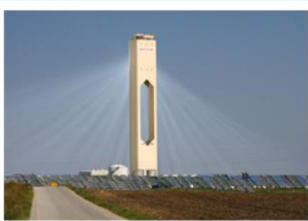
concentrating solar system
