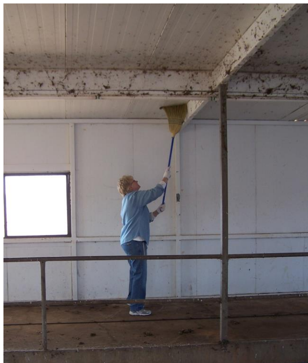
Debbie Toeplitz brushes cobwebs from the ceiling.
