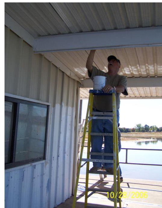
Joe Rostochil paints ceiling beams.
