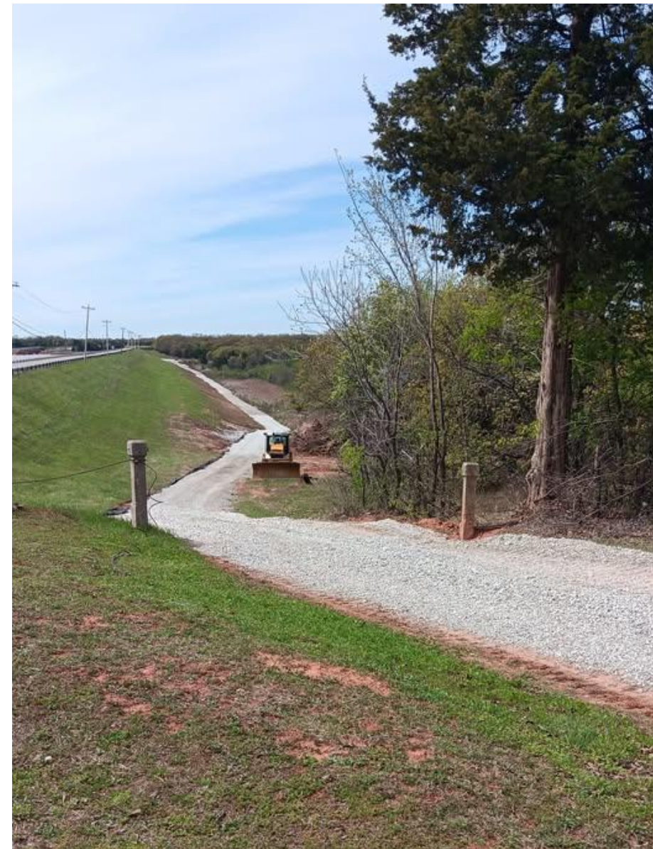
Road Added for Maintenance
