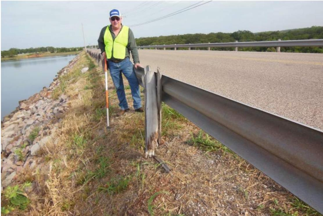
Photo No. 12: View of damage to guard rail post on the upstream side of the road.
