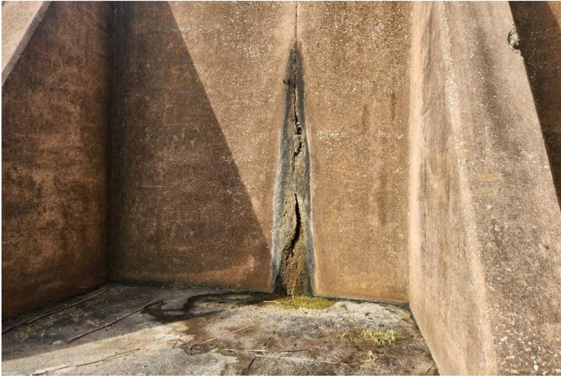
Photo No. 28: Some cracking and spalling along a concrete joint in one of the flip buckets.
