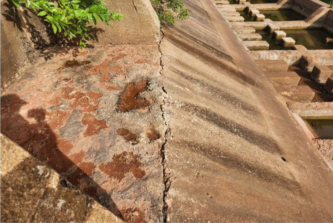
Photo No. 30: View of a concrete joint and some woody debris in the stilling basin.
