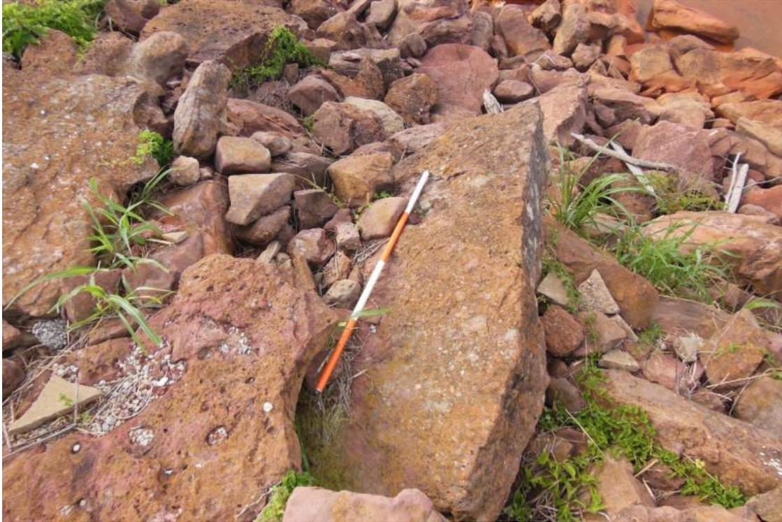
Photo No. 6: View of riprap on the upstream slope. Notice the mismatched sizes of rock and large sandstone slabs. The scale rod shown is 4ft long.
