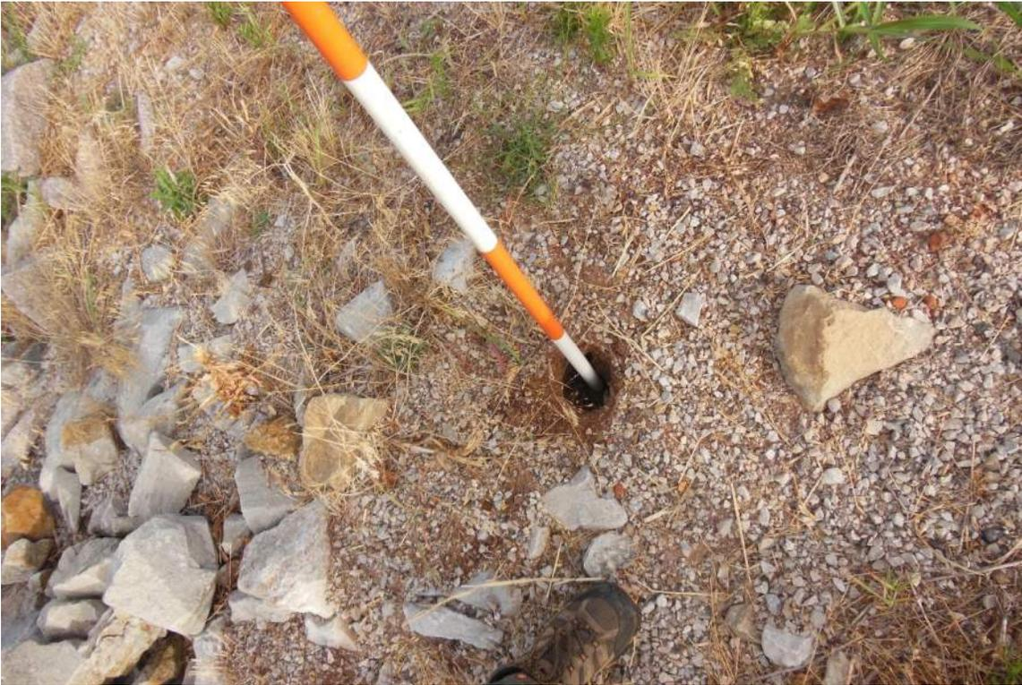
Photo No. 8: View of rodent hole on the upstream slope.
