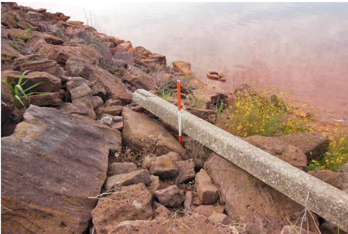
Photo No. 5: Photo of a large piece of concrete debris on the upstream slope. Rod is shown for scale.
