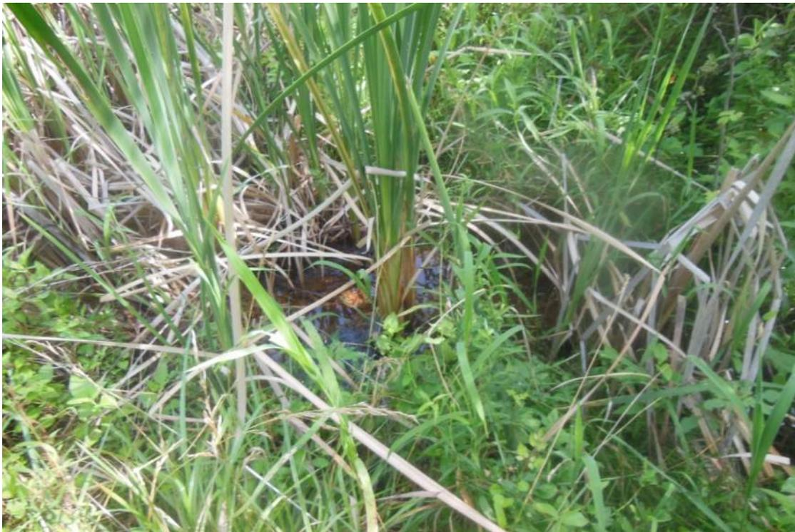
Photo No. 19: Typical view of standing water from seepage on the downstream toe near the abutments. The water was mostly clear and not visibly flowing.
