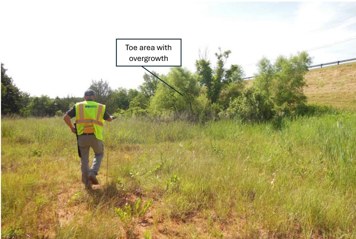
Photo No. 17: View of the downstream toe just east of the spillway. Notice the overgrowth along the toe.
