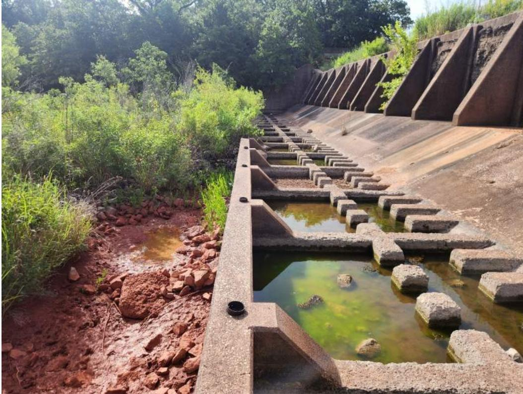
Photo No. 32: Downstream side of stilling basin structure. Some displaced riprap from previous flows noted downstream of end sill. Concrete surface weathering on energy dissipators.
