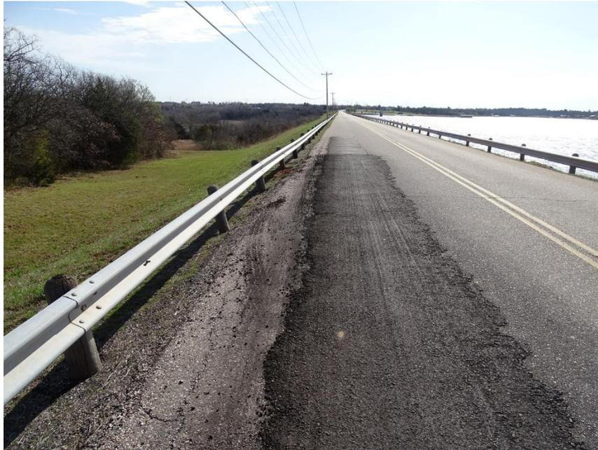
**Figure 11. Road Repairs noted during the July 2024 inspection by FNI**
