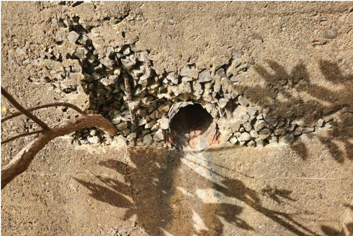
Photo No. 29: View of honeycombed concrete at base of back wall of flip bucket.
