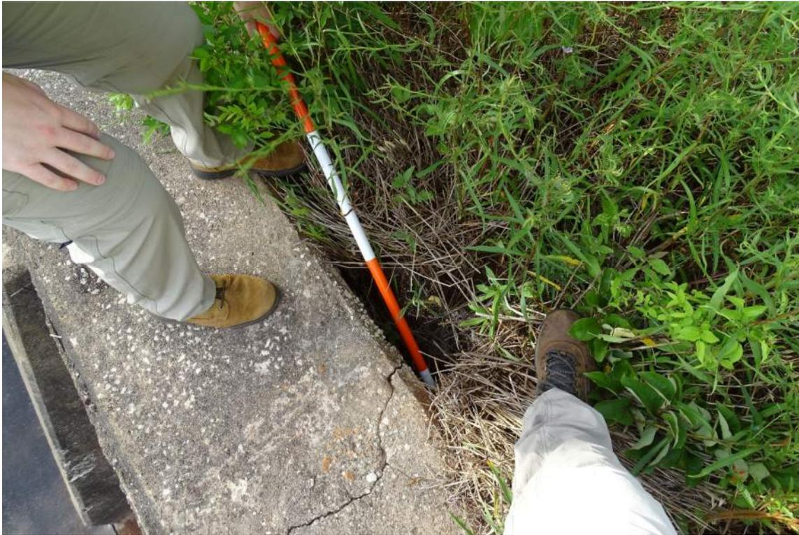
Photo No. 26: Additional scour upstream of the flip bucket walls.
