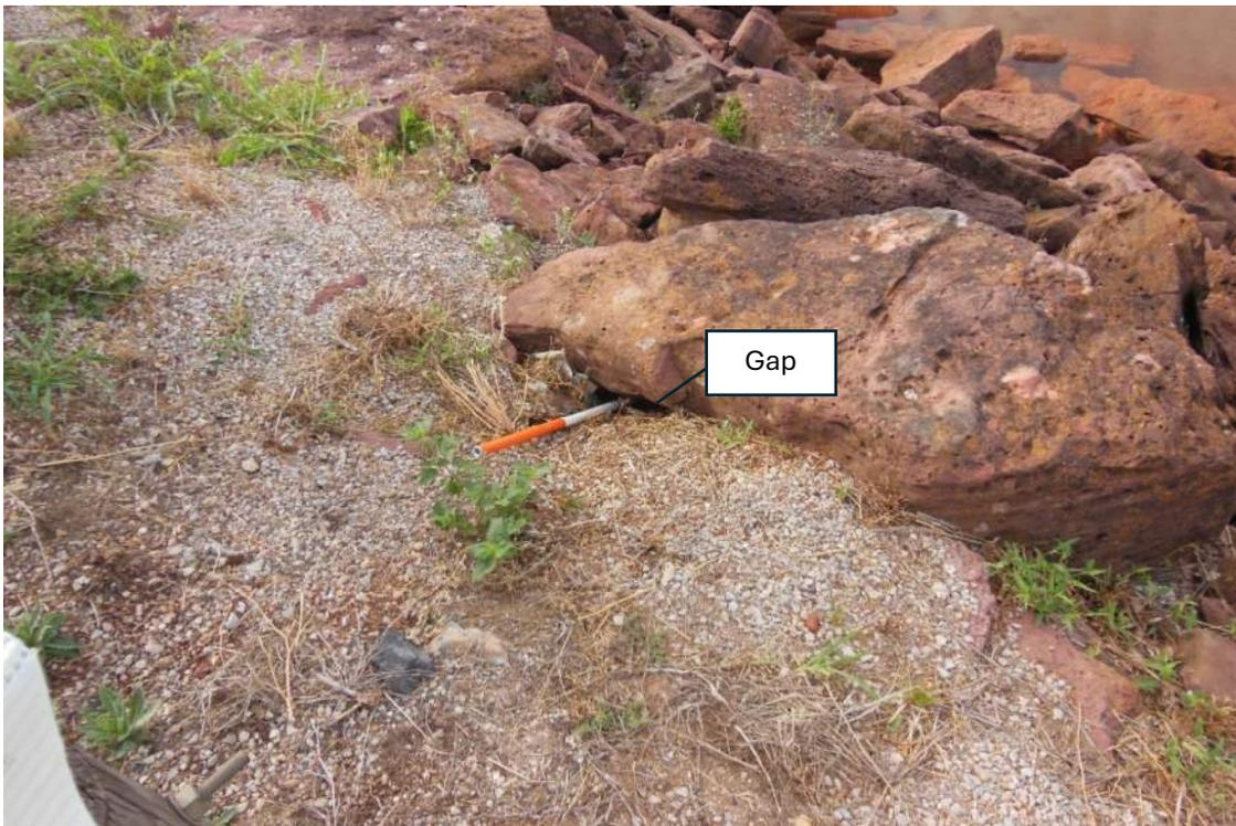
Photo No. 7: View of a gap under a large sandstone boulder near the crest of the slope. The gap has been created from washout of finer material under the large riprap.
