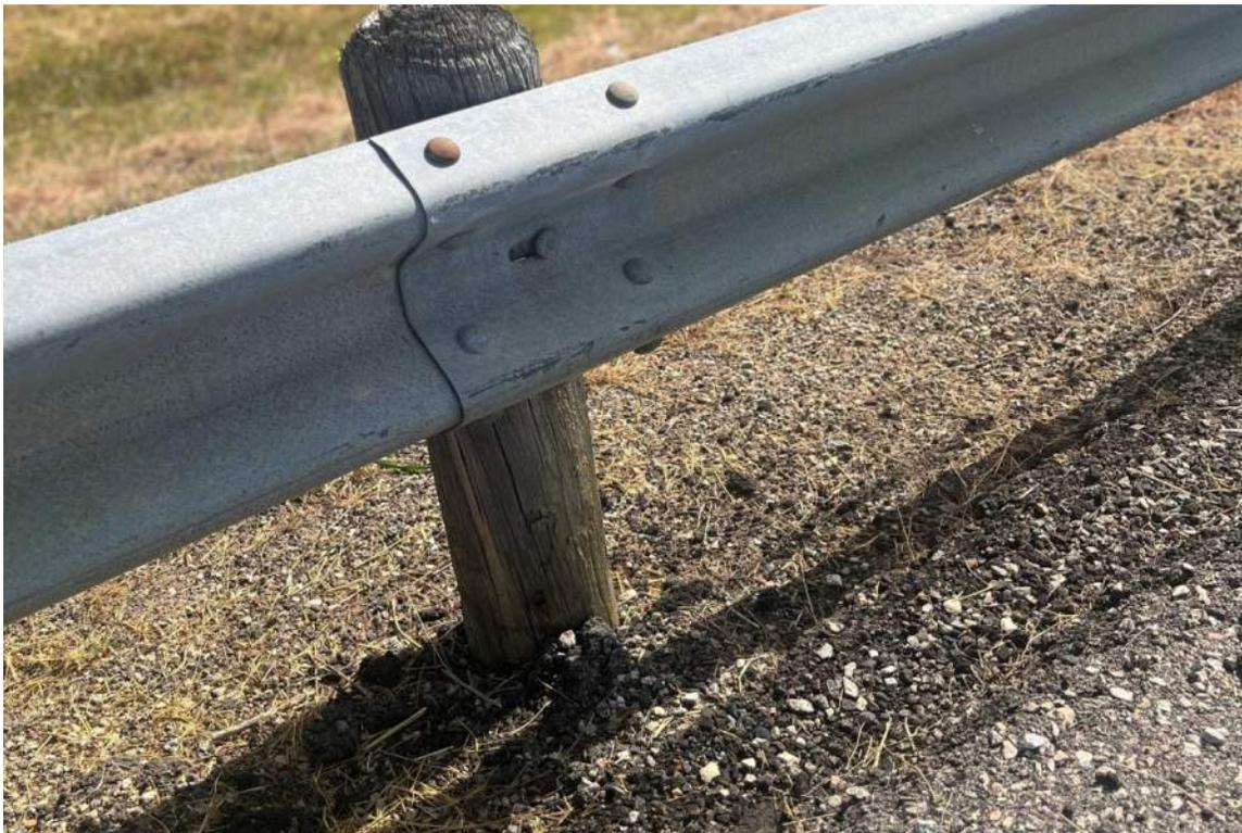
Photo No. 2: View of minor damage to guard rail along the crest of dam.
