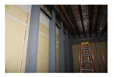
Close up view of 12" steel I-beams that are anchored in concrete at the bottom and bolted to the steel support for the floor on the second level. A stable grouting material is used to seal the I-beams to the wall.
