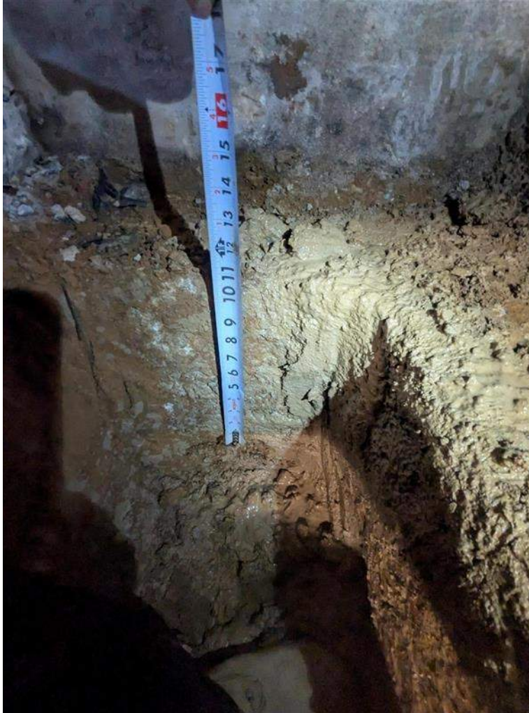
Photo 3: Interior Test Pit TP-1A; view of foundation thickness
