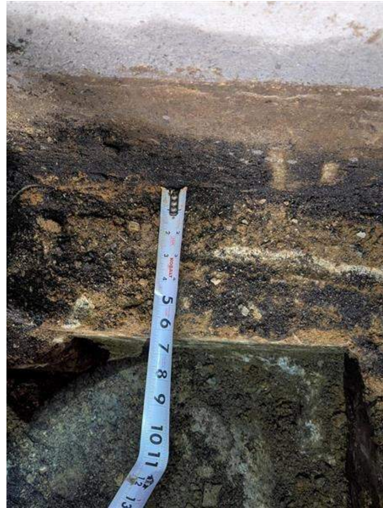
Photo 16: Interior Test Pit TP-4A; view of foundation projection after stepdown
