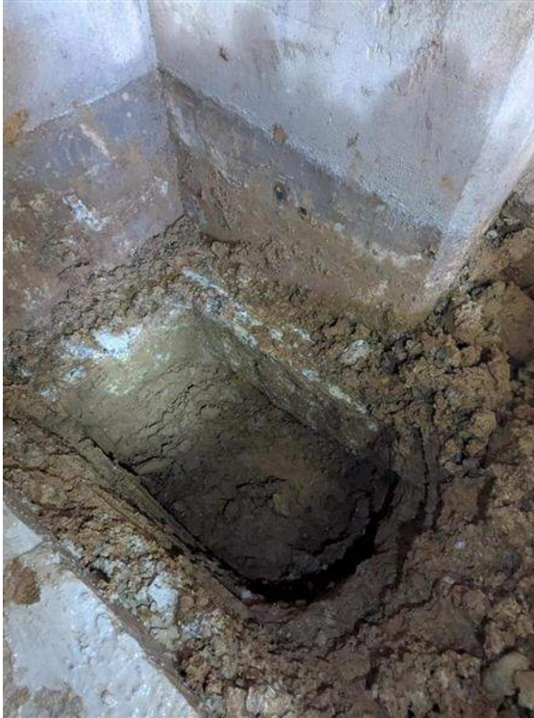
Photo 5: Interior Test Pit TP-2A (away bleachers). Floor slab and foundation exposed
