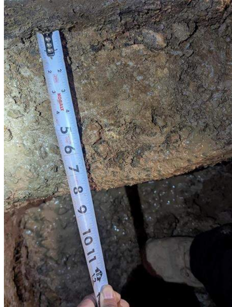
Photo 4: Interior Test Pit TP-1A; view of foundation projection
