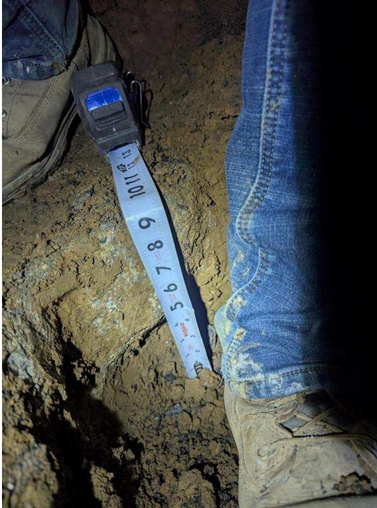
Photo 11: Interior Test Pit TP-3A; view of foundation thickness
