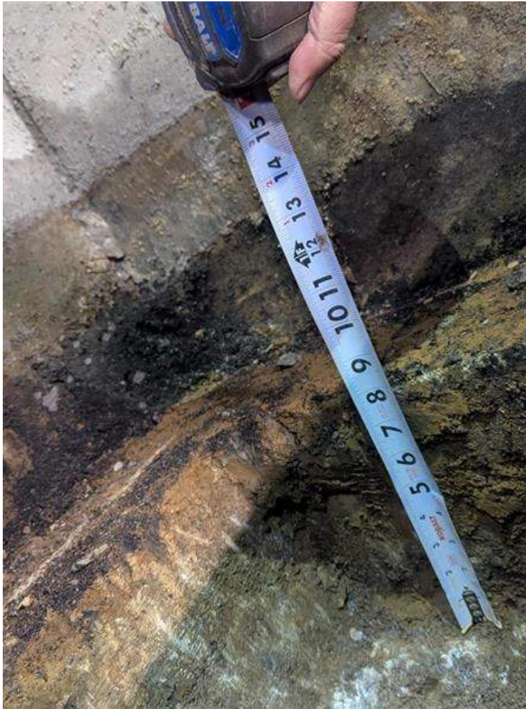
Photo 15: Interior Test Pit TP-4A; view of foundation thickness after stepdown
