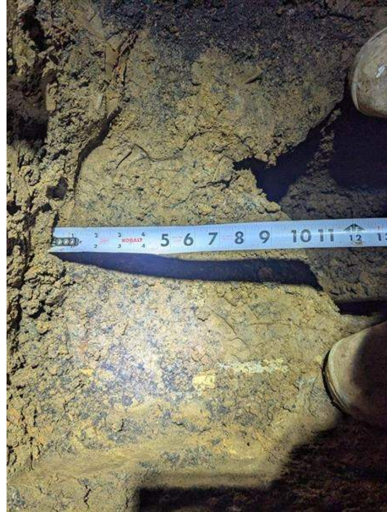
Photo 12: Interior Test Pit TP-3A; view of foundation projection
