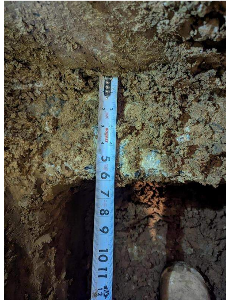
Photo 8: Interior Test Pit TP-2A; view of foundation projection
