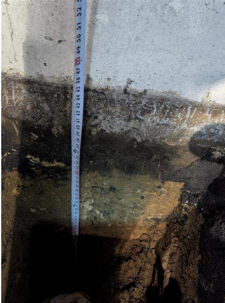
Photo 9: Interior Test Pit TP-3A (home bleachers). Floor slab and foundation exposed
