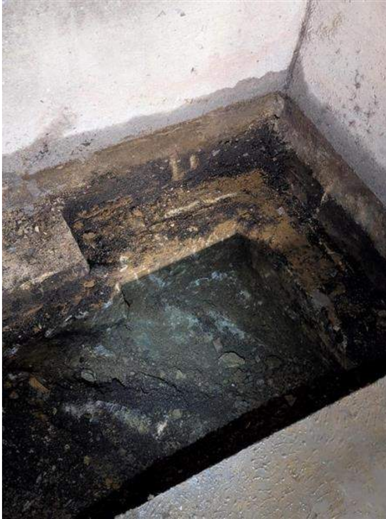
Photo 13: Interior Test Pit TP-4A (home bleachers). Floor slab and foundation exposed
