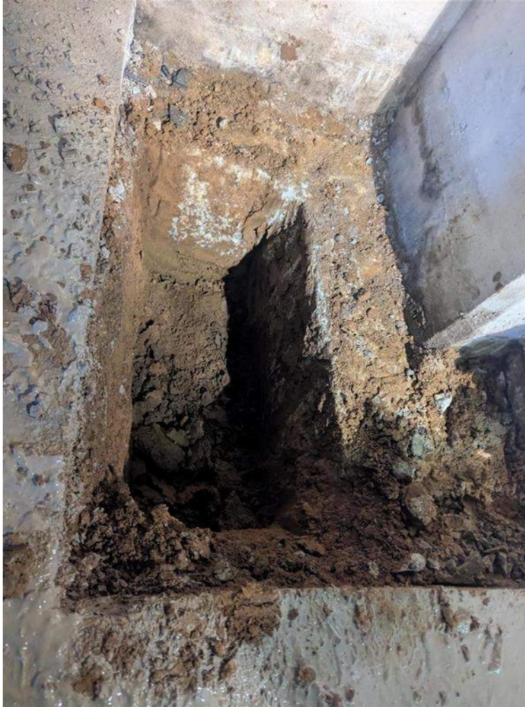
Photo 1: Interior Test Pit TP-1A (away bleachers). Floor slab and foundation exposed
