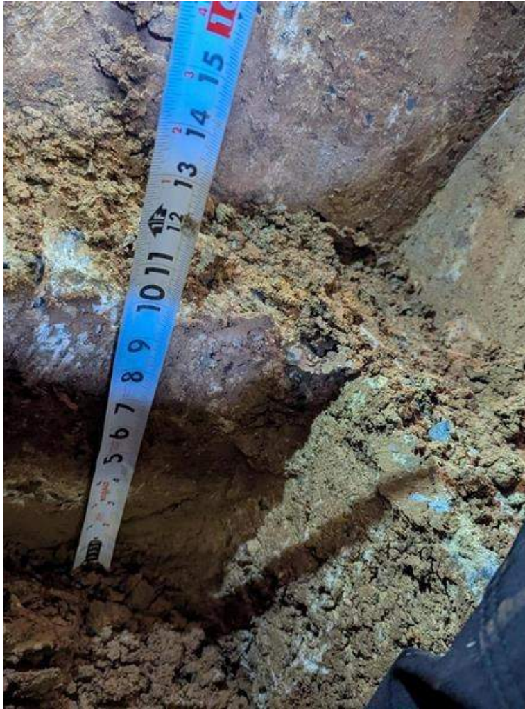
Photo 7: Interior Test Pit TP-2A; view of foundation thickness
