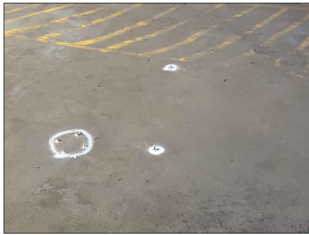
IMAGE 1: CUT STEEL DOWELS FLUSH WITH CONCRETE FLOOR. GRIND SMOOTH AS REQUIRED. TYP THROUGHOUT BUILDING
