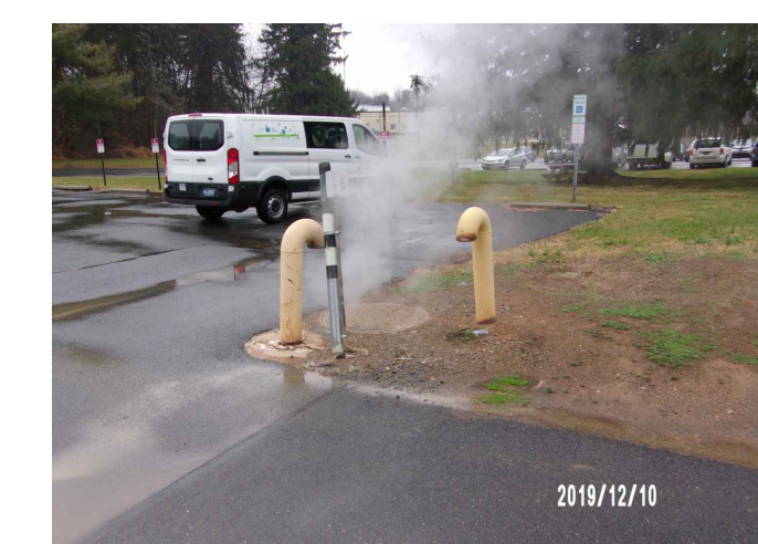
6 DEMO STEAM MANHOLE MH-6 Scale: NONE
