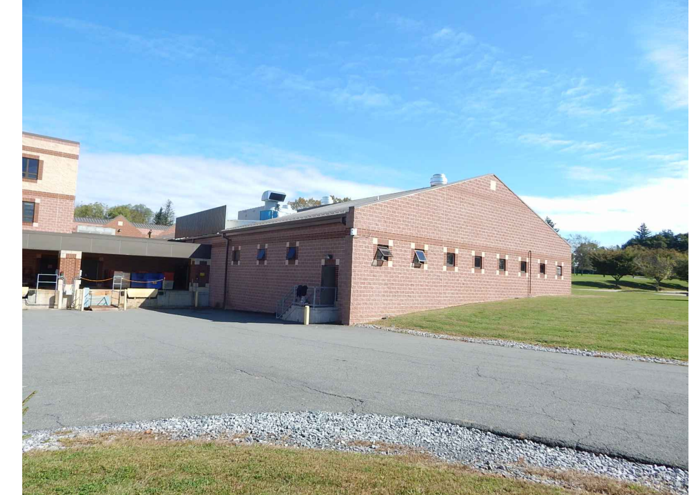
2 EXISTING BUILDING PHOTO Scale: NONE
