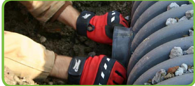
INSERTA TEE CONNECTION DETAIL
