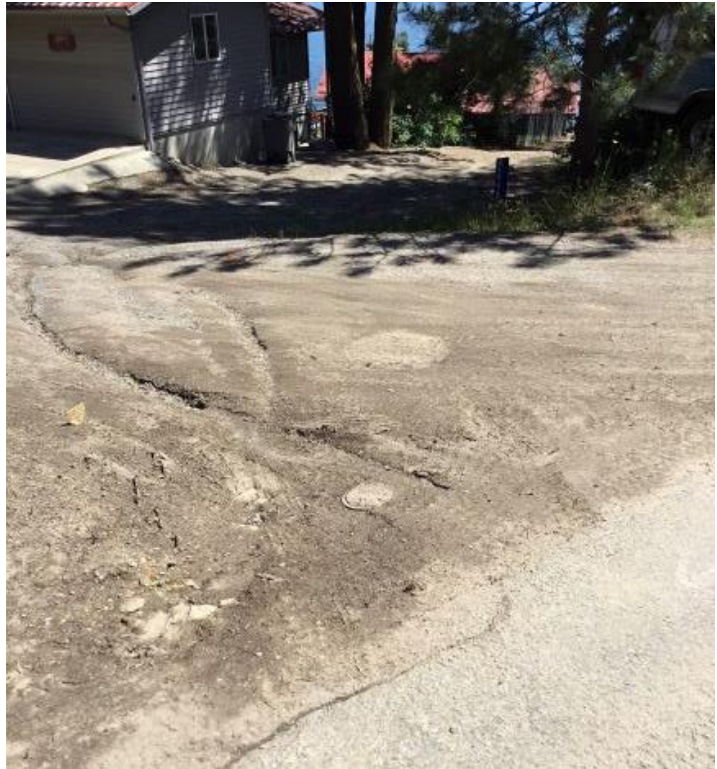
The water damage and erosion caused by the May 30 th thunderstorm flowing down road 1 and into the Absolonson's driveway.
