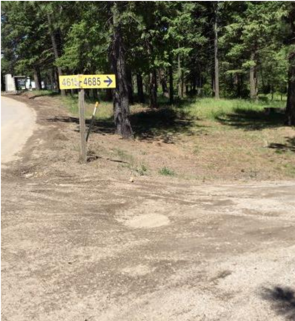
S. Loon Lake Rd – LSH Road 1 Entrance. There is sewer (large circle), gas line and communications lines running down the road
