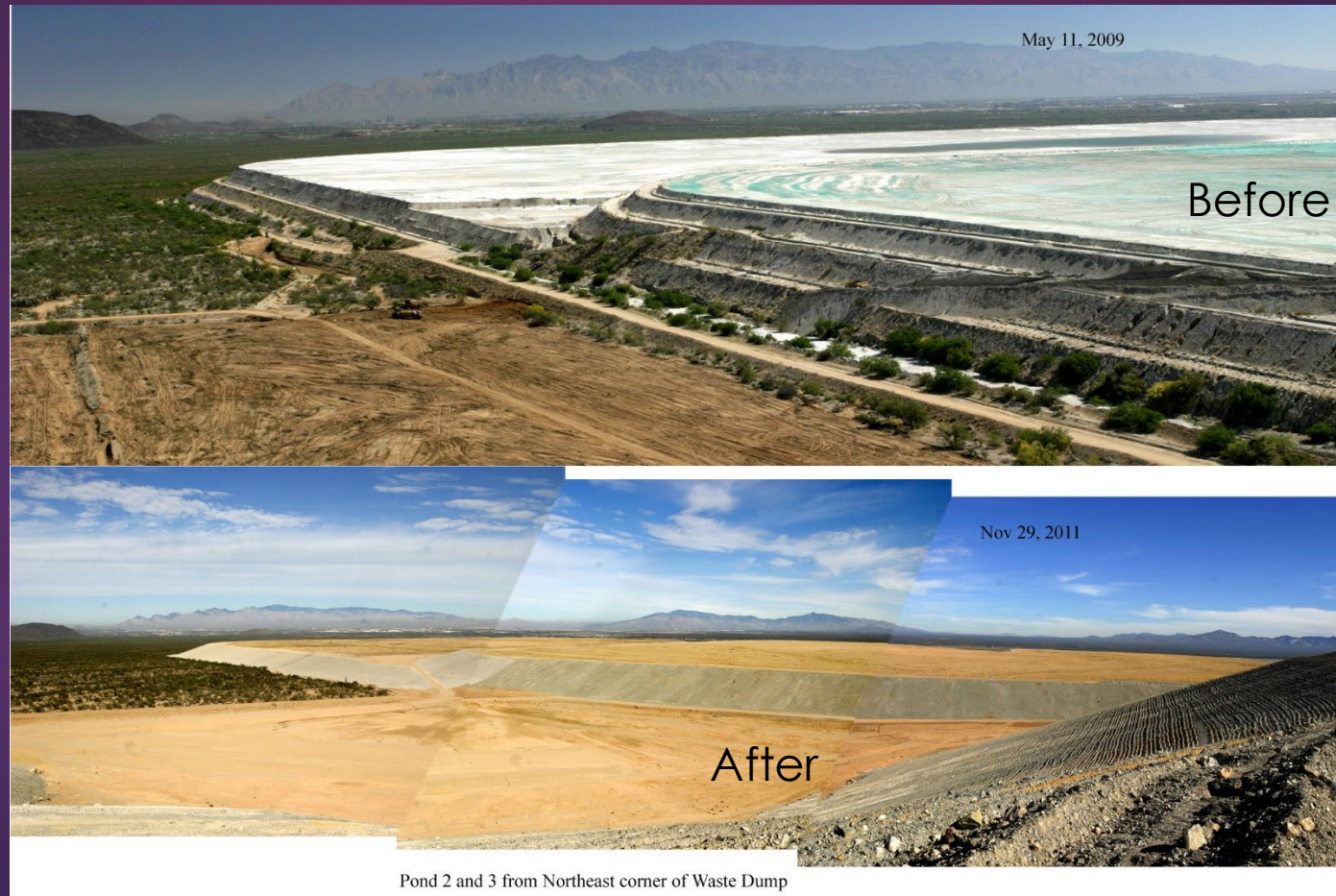
TAILINGS PONDS 2 & 3 FROM NORTH DUMP
