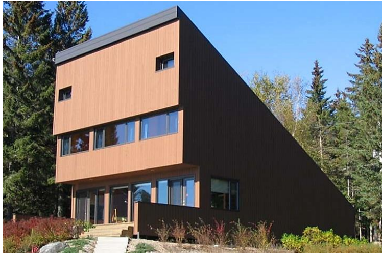
Straight South cantilevering to reduce solar radiation in the Summer and welcome it in the Winter
