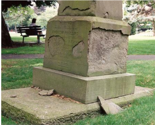
Example of soluble salt damage to a headstone in the form of spalling.
