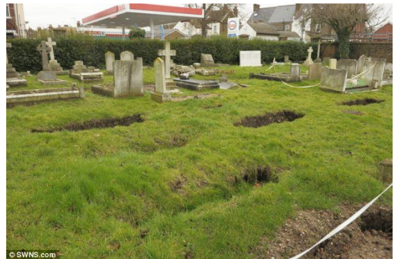
An extreme example of ground settlement on graves.
