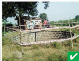
Open wells with fence
