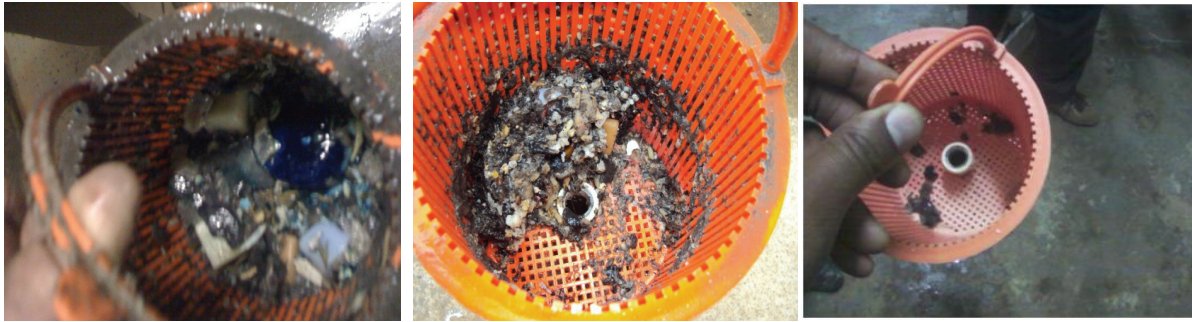
Figure 20. The sieves a few days before the awareness session (Left); after the awareness session (Centre); and after disconnecting the laboratory basins (Right)
