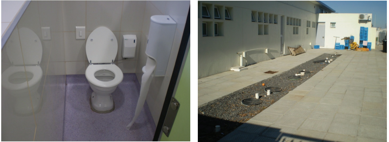
Figure 7. (Left) One of the centre's toilets reusing greywater for flushing. (Right) Several submerged filters and tanks that house the pumps that convey greywater to the toilet bowls
