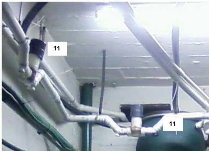
Figure 21. Inline chlorinators installed to improve disinfection of the greywater
