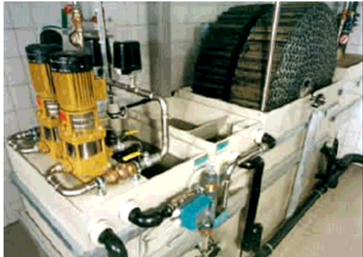
Fig. 5: Multi-stage Rotating biological contactor (RBC) for greywater recycling.
