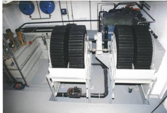
Fig. 5: Multi-stage Rotating biological contactor (RBC) for greywater recycling.
