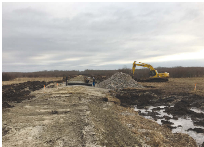
SRRCD staff assisting contractors with the installation of cell grid and geotextile matting
