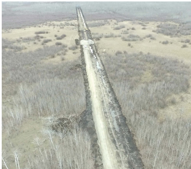
Aerial photo of Penner Water Retention Project
