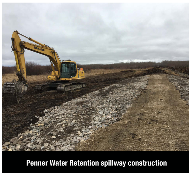
SRRCD staff assisting contractors with the installation of cell grid and geotextile matting
