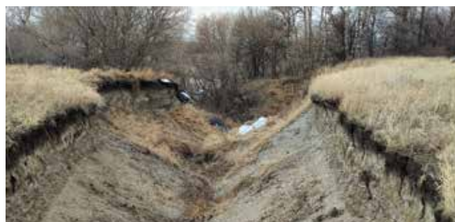
Repairing gullies to assist in improving drainage.
