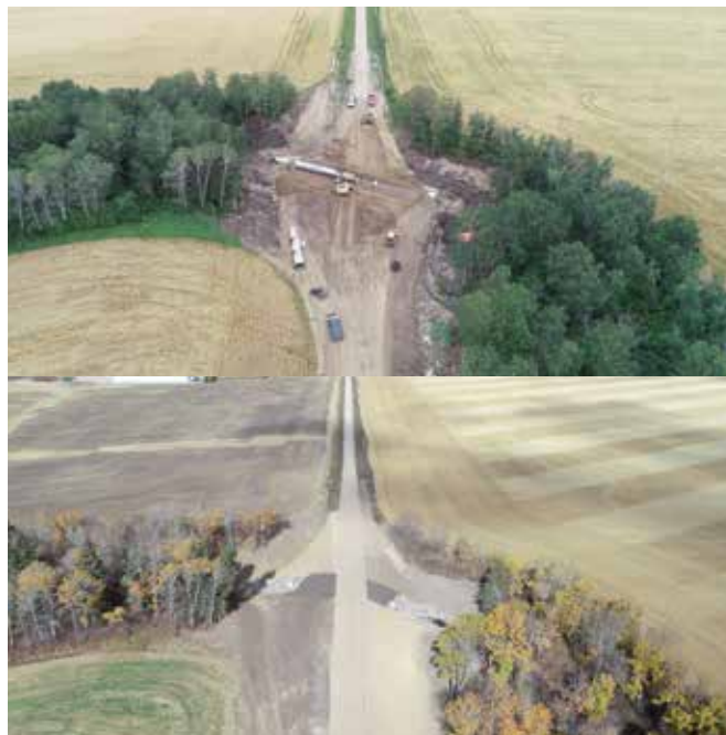
Miller Retention structure - flood and erosion control with water retention.
