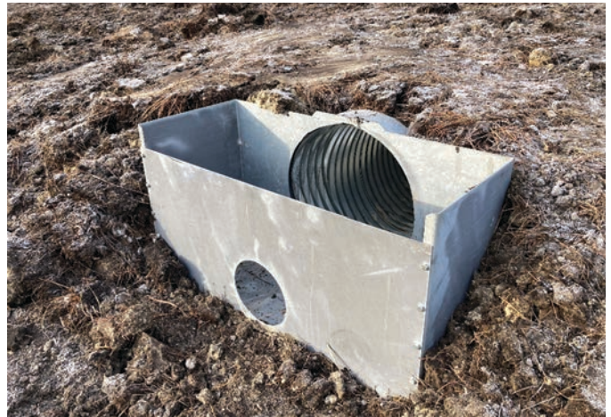
Culvert control structure
