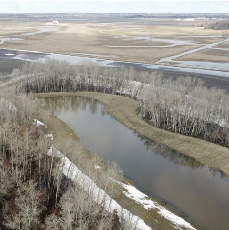
Ste Genevieve Water Retention Site
