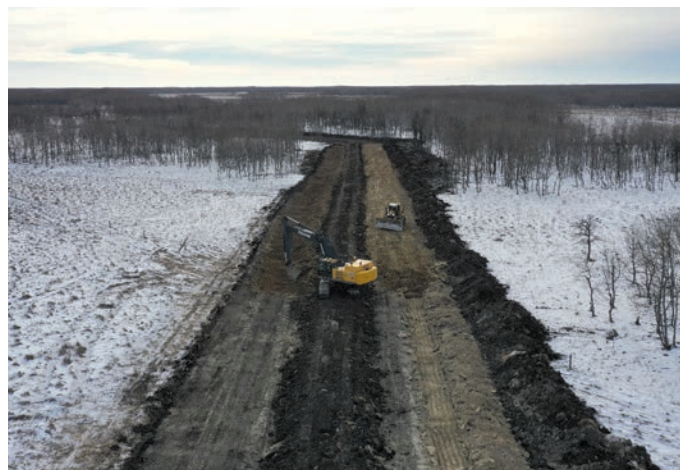
Construction of berm
