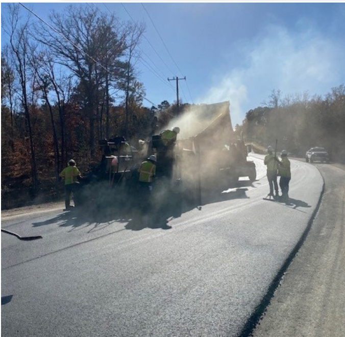
Fig. 2: Crews recently paved the new roadway
