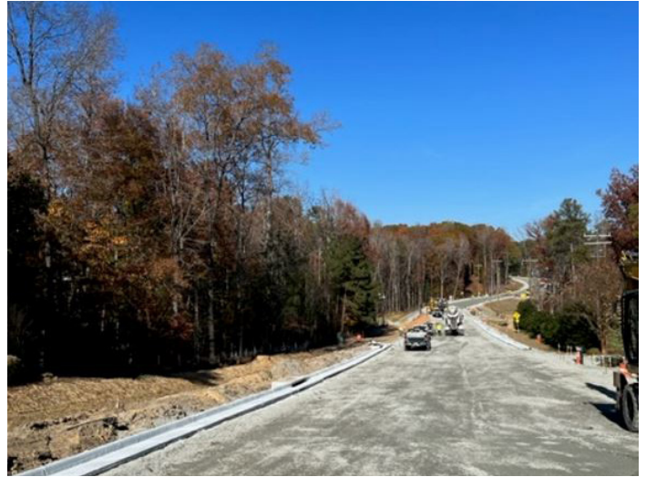
Fig. 1: Curb and gutter work was recently completed
