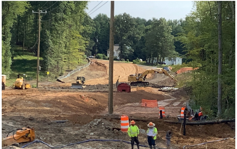
Fig. 1: Roadway Grading and Embankment Fill
