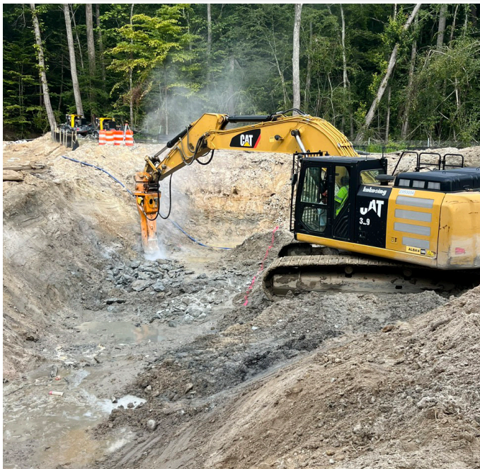
Fig. 2: Rock Demolition at Abutment B Footing
