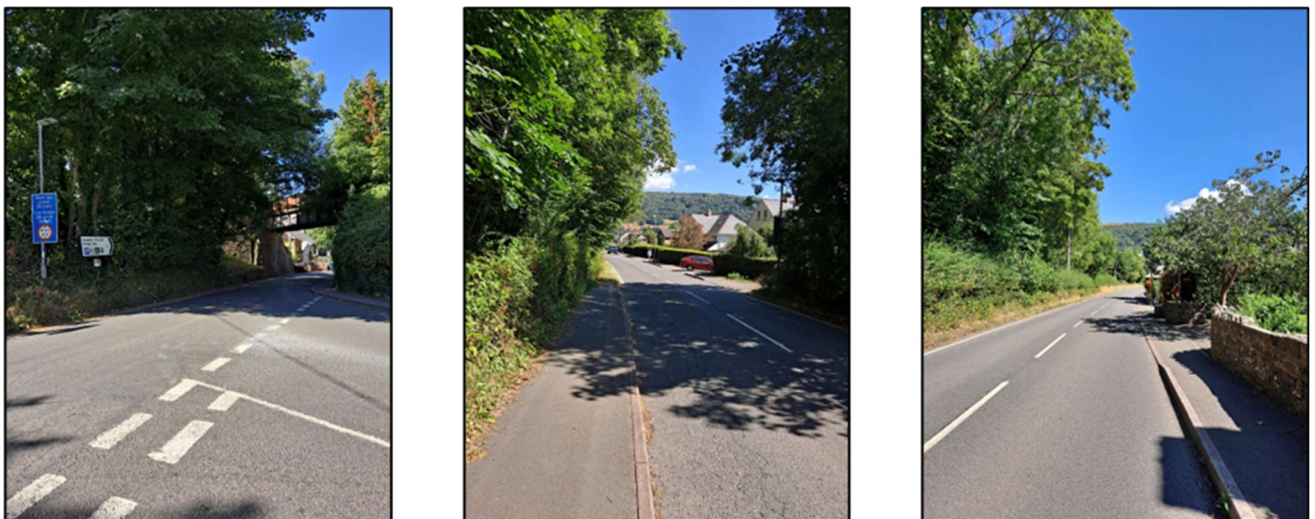
Figure 6 – Footway Provision, Station Road
