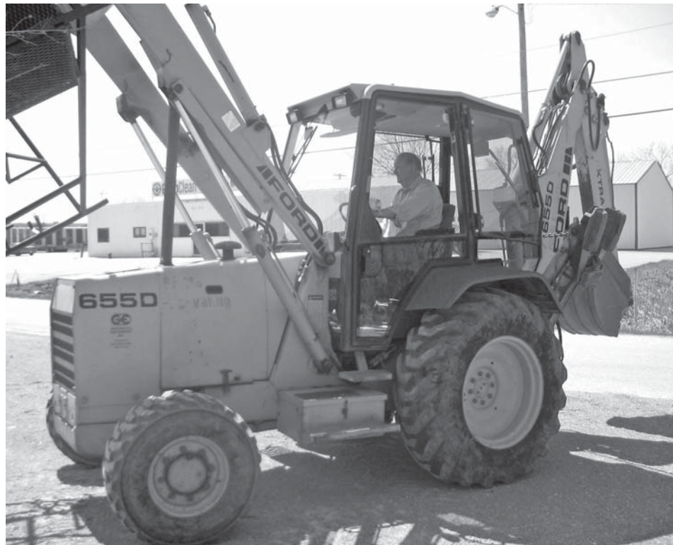
Besides running his dealership in Oshkosh, Mueller likes to drive a backhoe and take the wheel when he digs footings, roads, and parking lots for his buildings and subdivisions.
