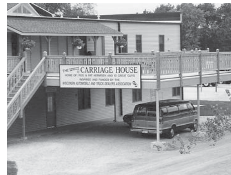
The WATDA Carriage House boys home at Rawhide Boys Ranch shortly after completion.
