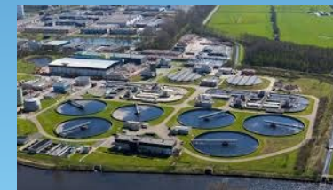
Sewage treatment plants
