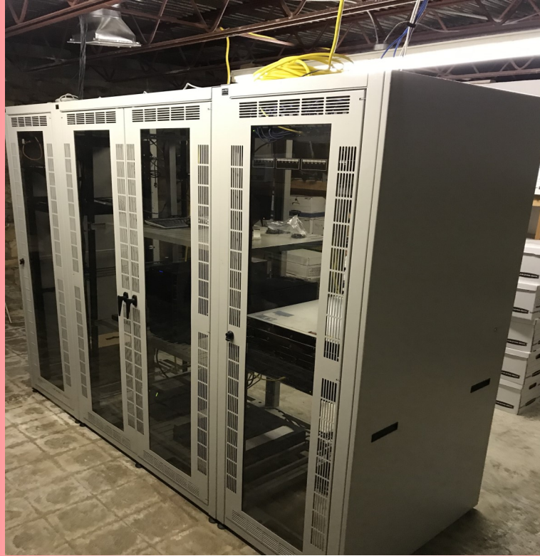
The centralized server and network cabinets store the phone system, internet routers, and servers for accounting systems and user storage.
