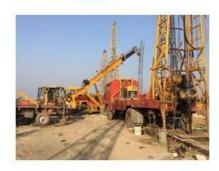
10 Sets of Mechanical Rigs for smaller dia piles like 0.350,0.450,0.600 & 0.750 meter dia
