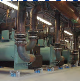
FLOOR MOUNTED ISOLATION
