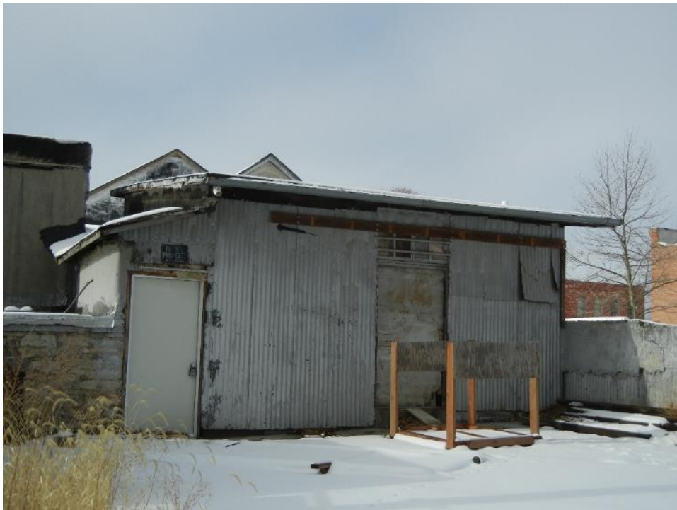
Photo 13: NE rear addition
