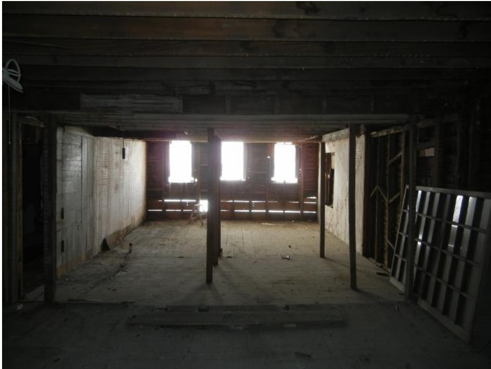
Photo 36: Second floor, north section, floor, storefront openings, loft framing
