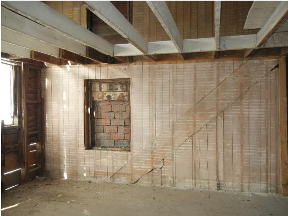
Photo 37: Second floor, north section, exterior opening (covered) and wall finish
