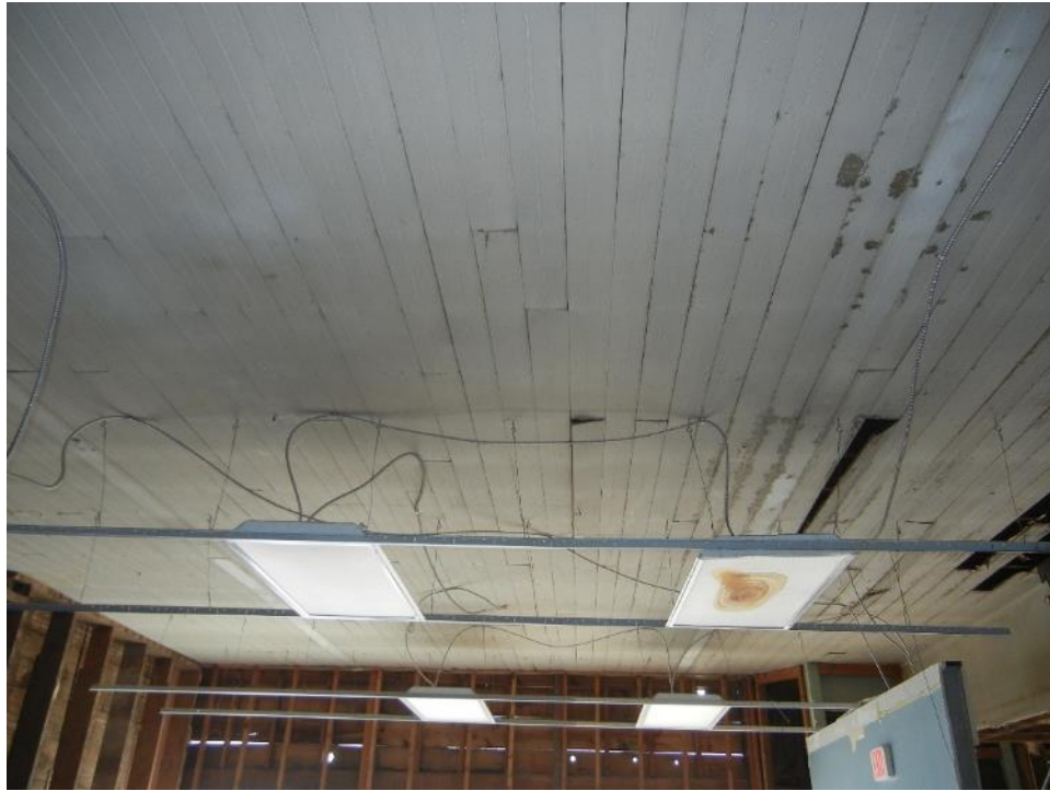
Photo 28: First floor, south section, ceiling
