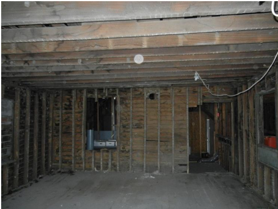
Photo 41: Second floor, north section, rear wall and ceiling joists
