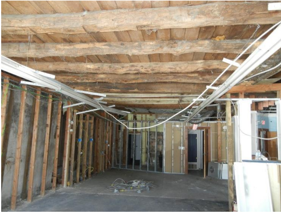
Photo 18: First floor, walls and ceiling, North section
