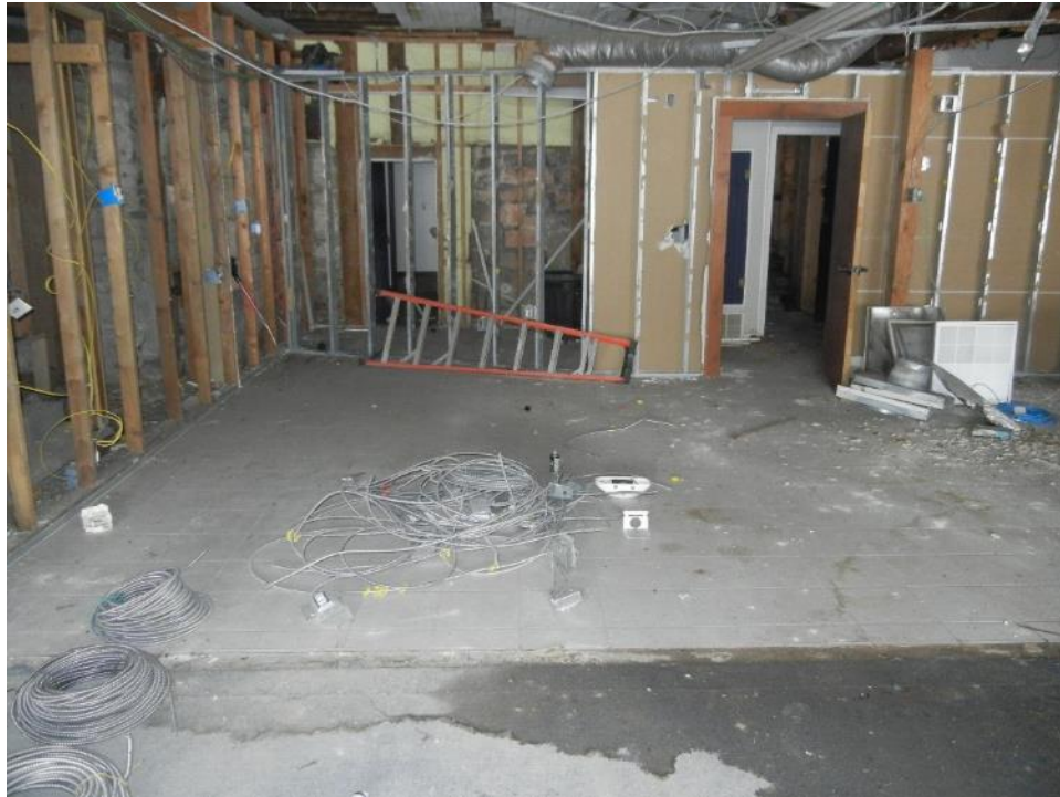
Photo 32: First floor, south section, south wall framing
