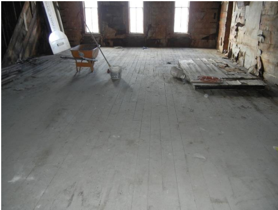
Photo 49: Second floor, south section, flooring and storefront windows
