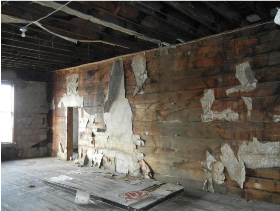
Photo 50: Second floor, south section, north wall sheathing (former exterior)
