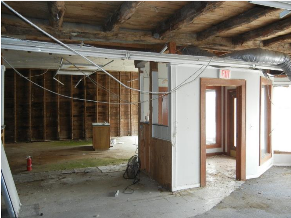
Photo 19: First floor, central entry framing, north ceiling, south wall
