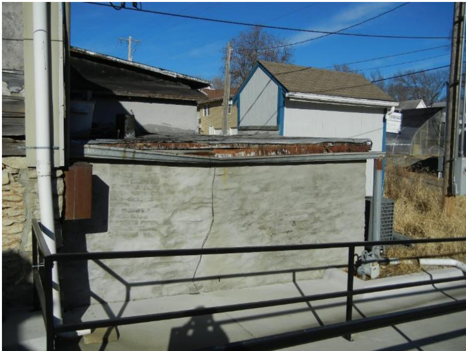
Photo 15: South section rear addition
