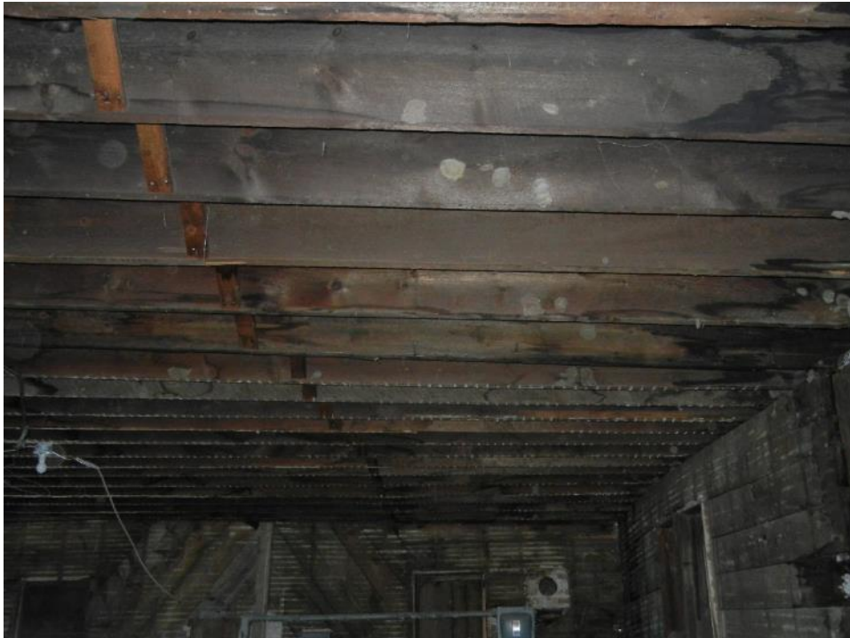
Photo 53: Second floor, south section, ceiling joists
