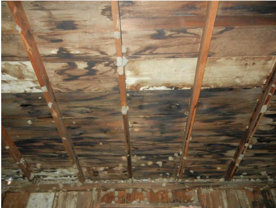
Photo 46: Second floor, north section, roof framing, second rear addition
