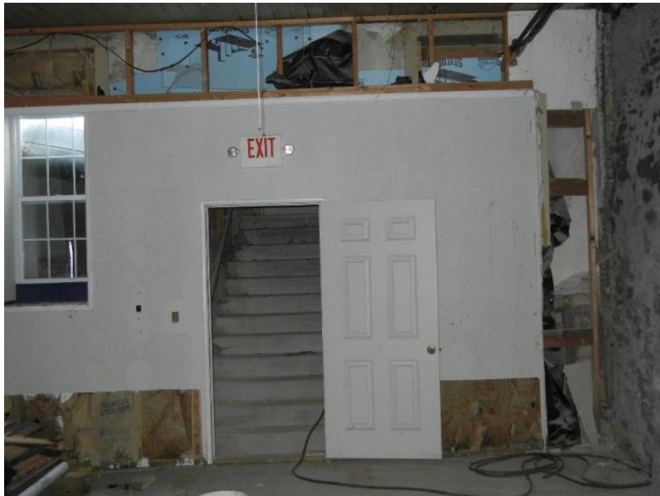
Photo 33: First floor, south section, rear partition and stair
