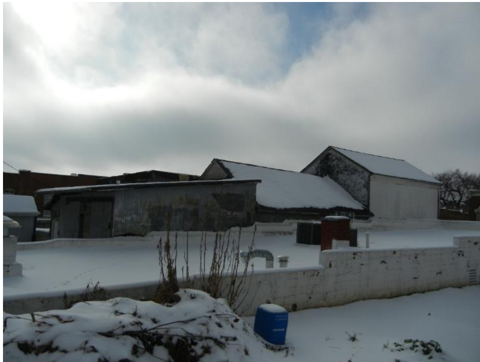
Photo 9: North elevation, three North sections
