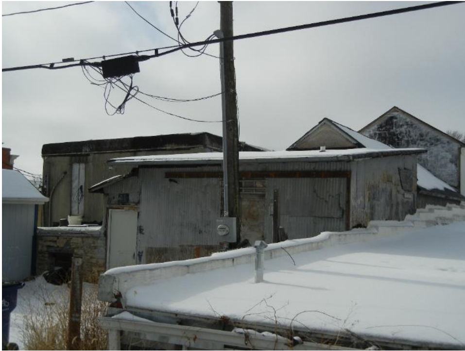
Photo 10: East elevation, rear addition
