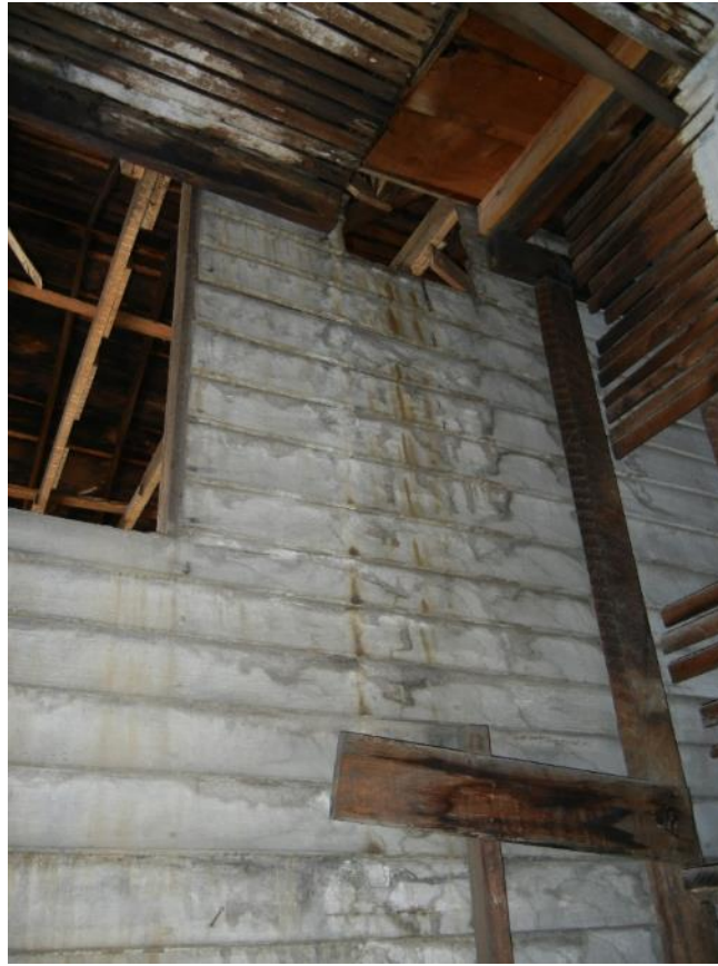
Photo 44: Second floor, north section, former rear exterior wall section
