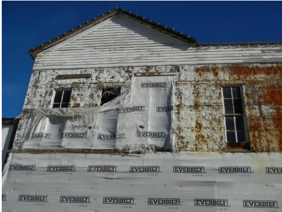
Photo 5: Detail of second floor storefront, north section
