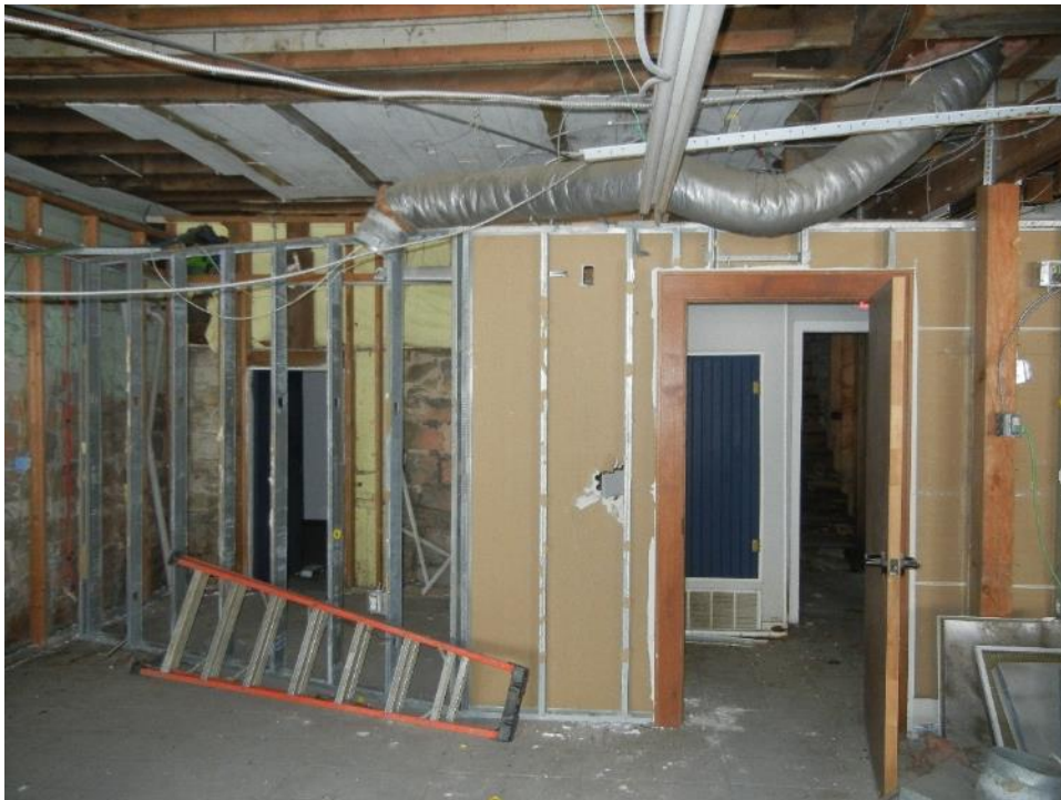
Photo 23: First floor, north section, east partition wall
