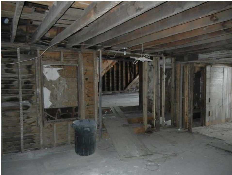
Photo 43: Second floor, north section, interior wall, opening, ceiling joists
