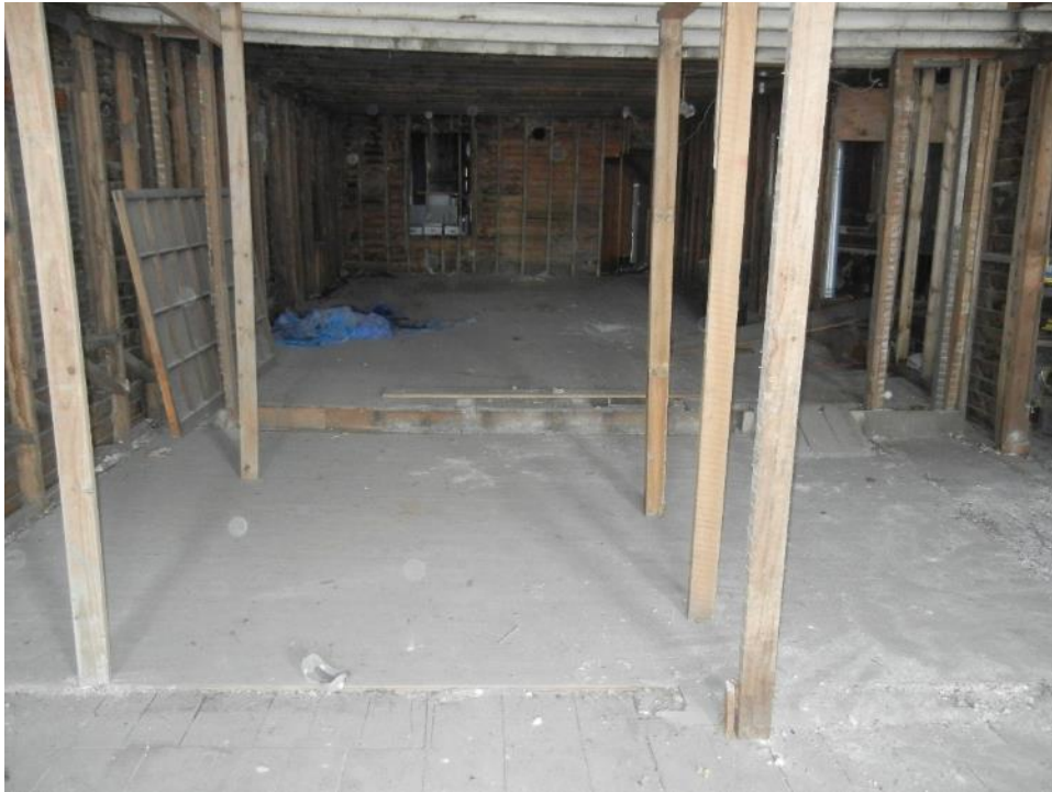
Photo 40: Second floor, north section, rear floor and rear wall framing
