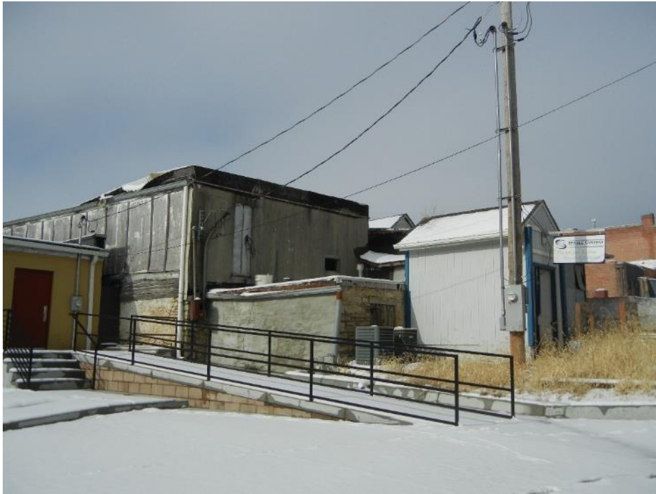
Photo 14: South section with additions
