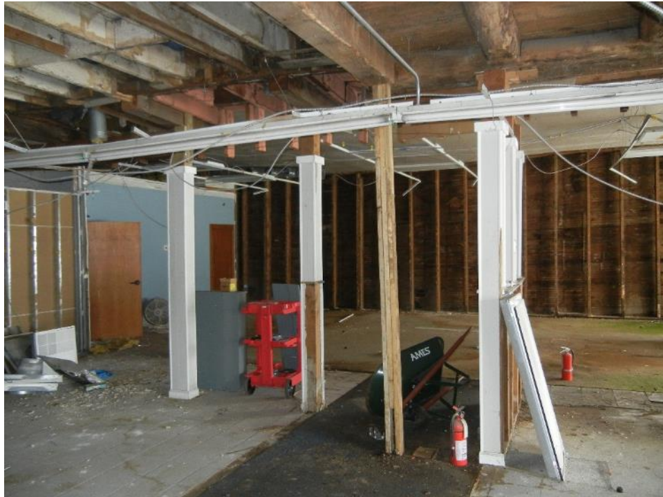
Photo 29: First floor, south section, partition posts, south and east walls
