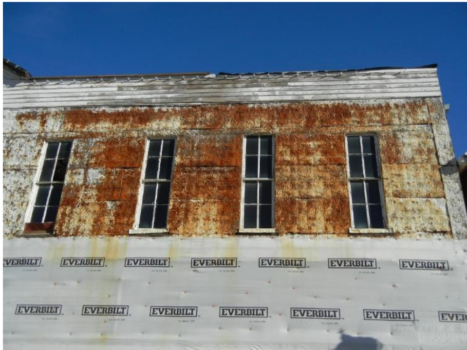
Photo 6: Detail of second floor storefront, south section
