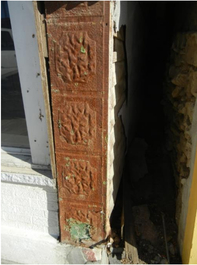
Photo 7: Detail of SW corner, pressed metal sheathing
