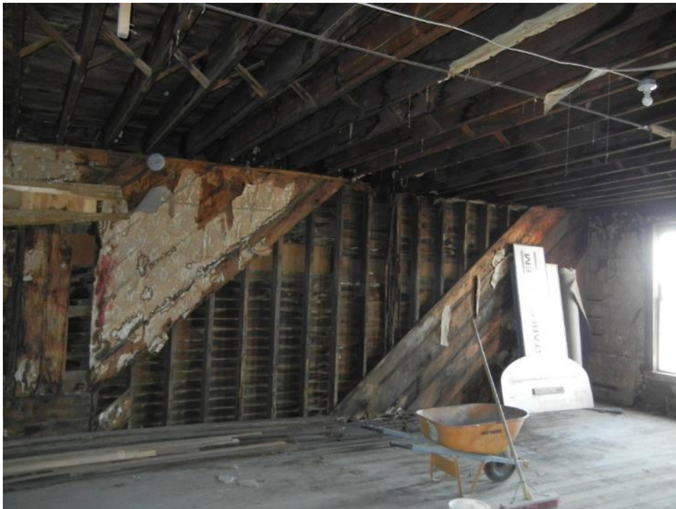
Photo 51: Second floor, south section, south wall sheathing and framing
