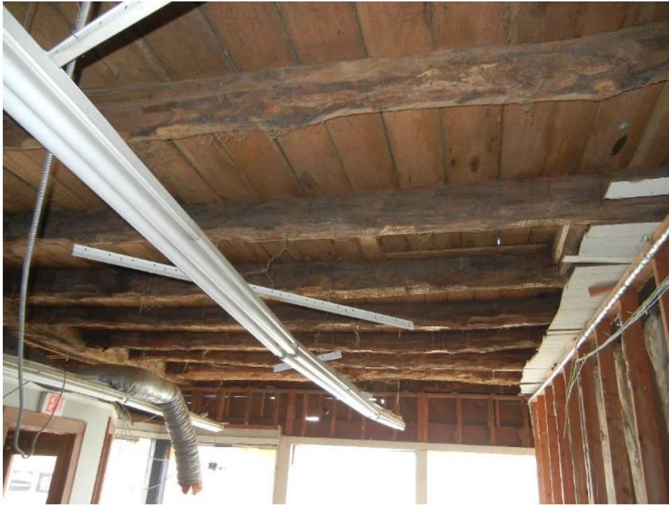
Photo 24: First floor, north section, ceiling framing
