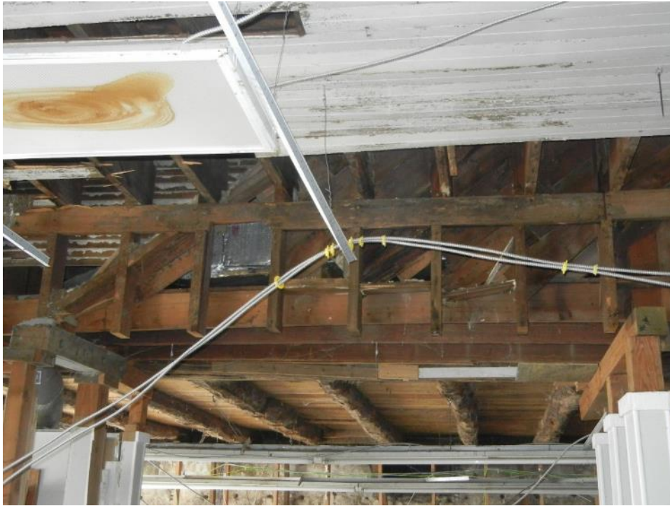
Photo 26: First floor, north section, ceiling and second story wall framing
