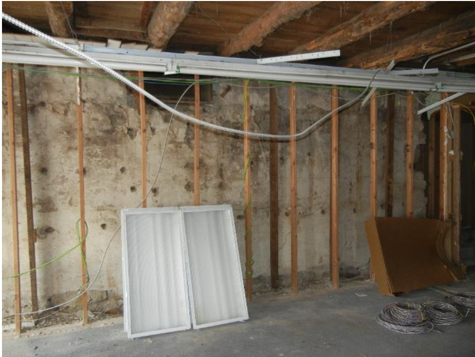
Photo 21: First floor, north section, north wall and ceiling
