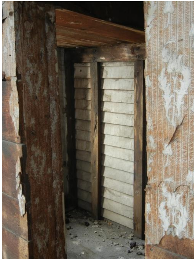
Photo 47: Second floor, north section, fragment of exterior weatherboard
