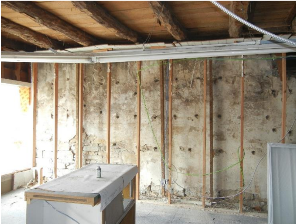
Photo 20: First floor, north section, north wall and ceiling
