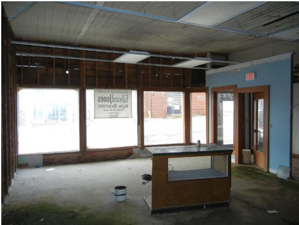
Photo 27: First floor, south section, storefront, ceiling, and entry wall
