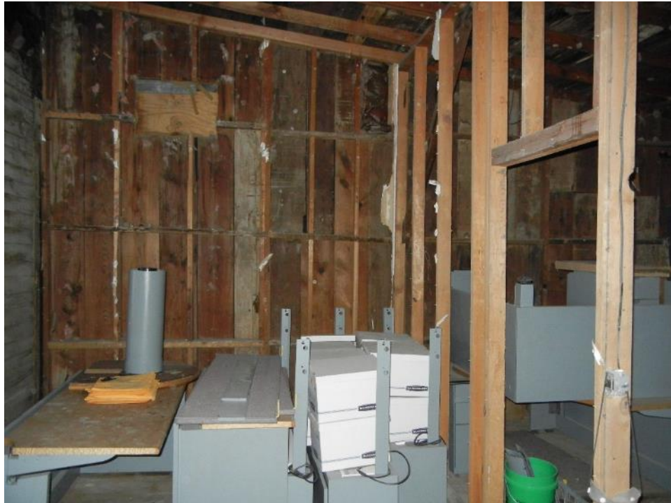
Photo 45: Second floor, north section, exterior framing, second rear addition
