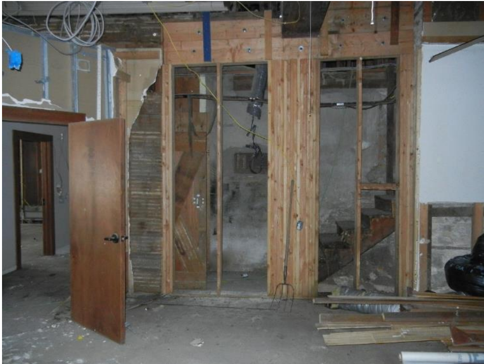
Photo 34: First floor, south section, partition with beam, rear stair
