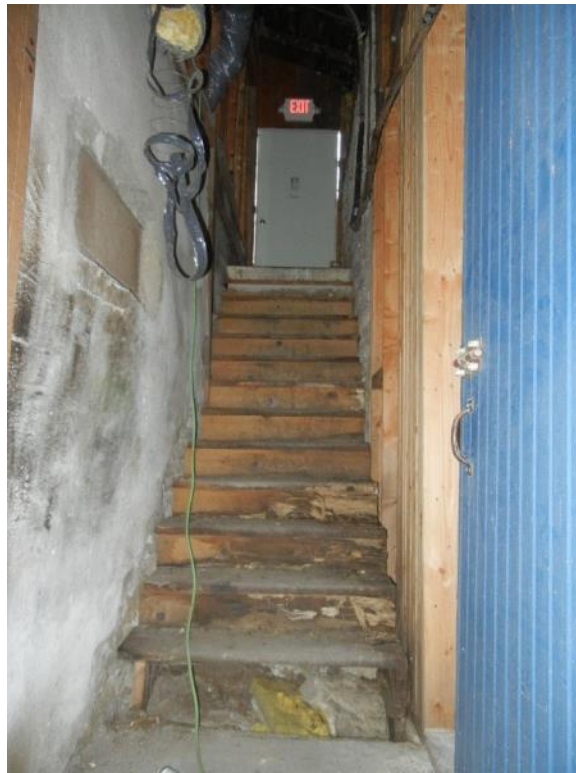
Photo 35: First floor, south section, stairway to rear entrance
