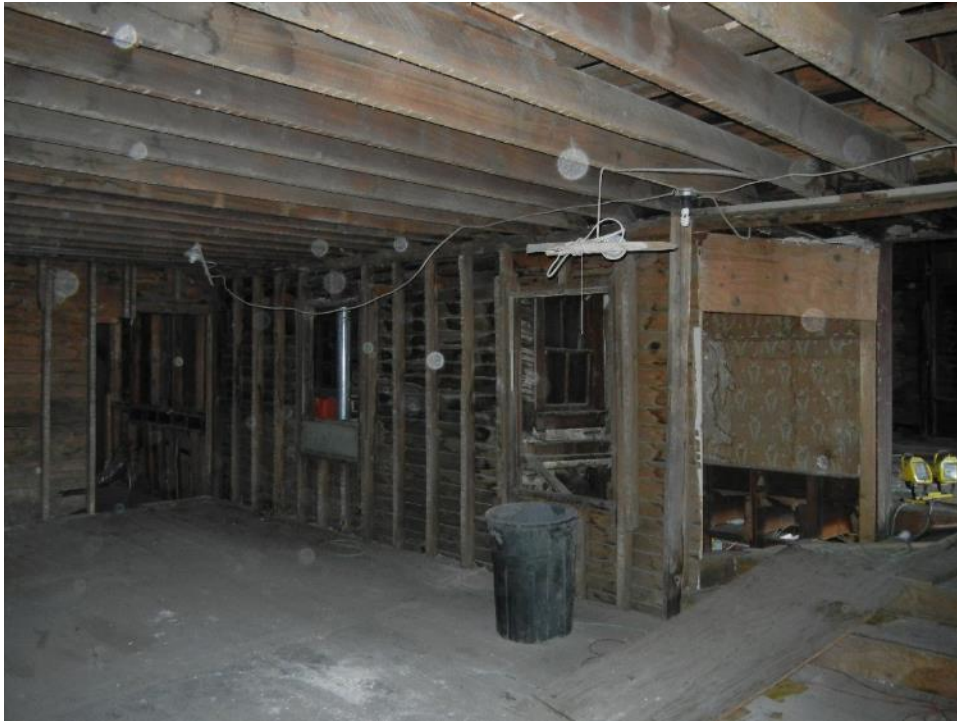
Photo 42: Second floor, north section, interior wall and ceiling joists
