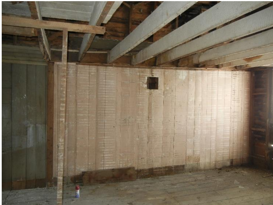
Photo 39: Second floor, north section, interior wall finish
