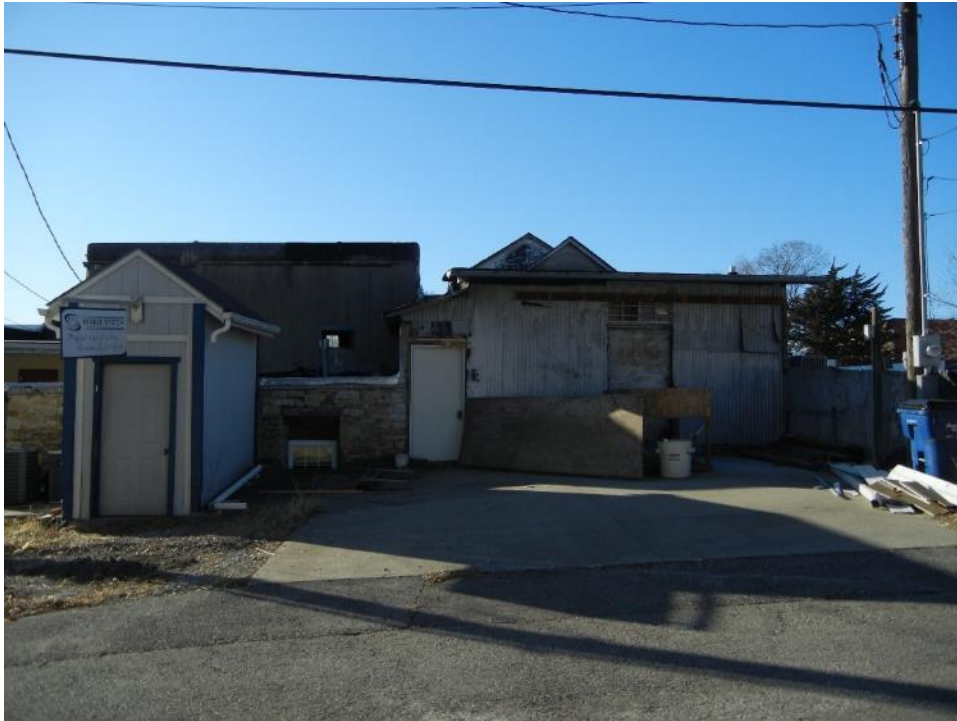
Photo 12: East elevation, additions
