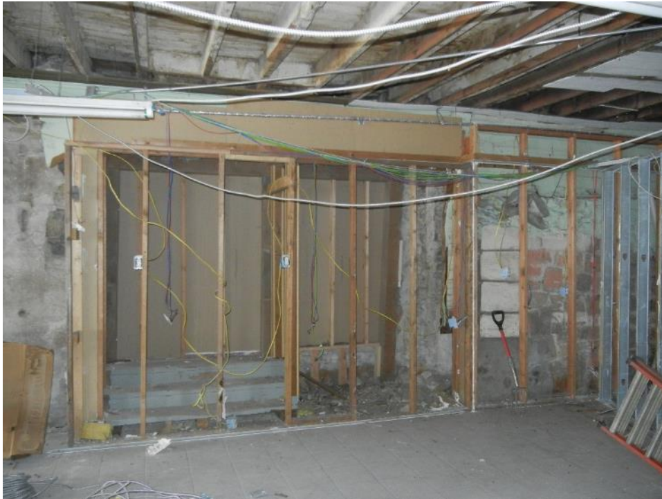
Photo 22: First floor, north section, north wall opening (covered)
