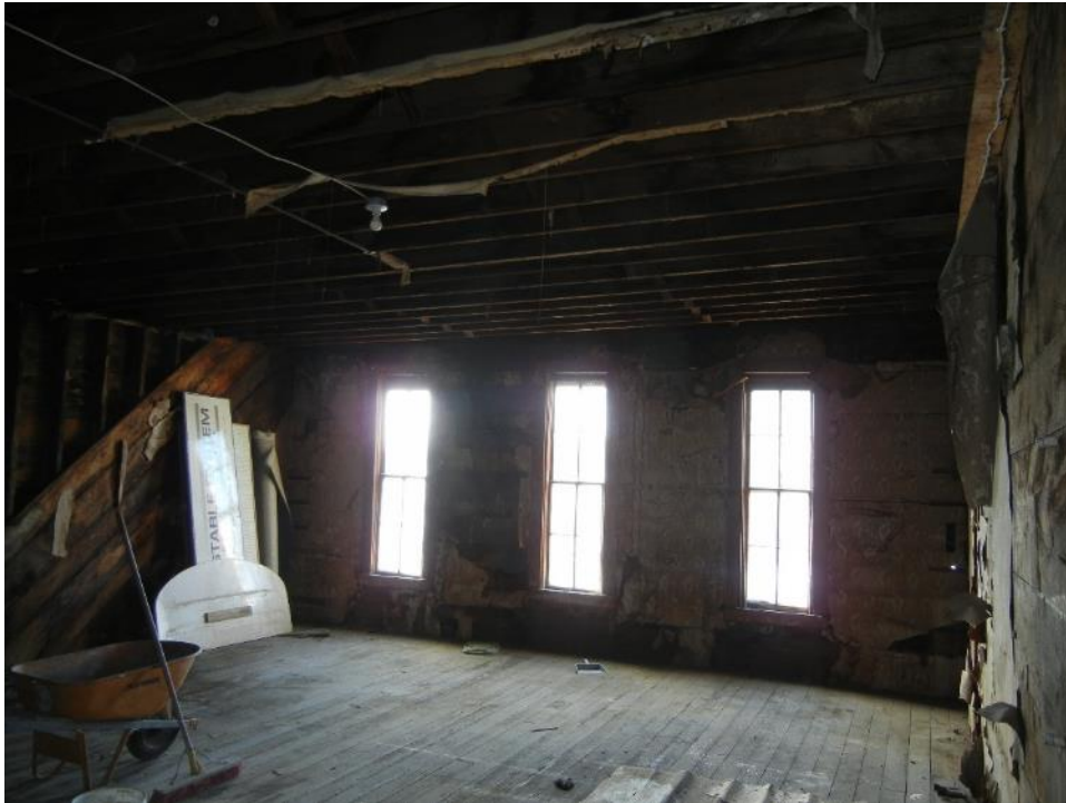
Photo 48: Second floor, south section, storefront windows and ceiling
