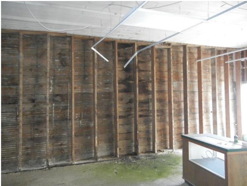
Photo 31: First floor, south section, east and south partition walls
