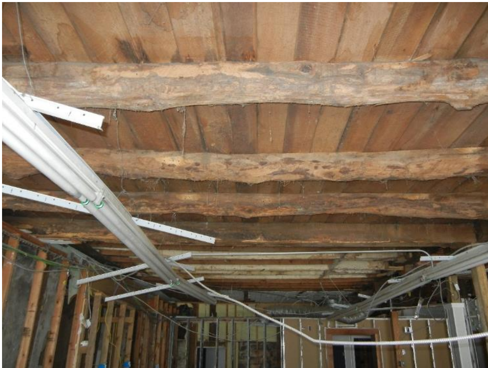
Photo 25: First floor, north section, ceiling framing
