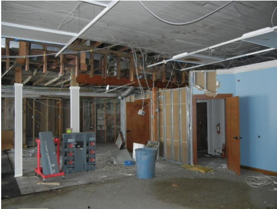
Photo 30: First floor, south section, partition posts, east partition wall
