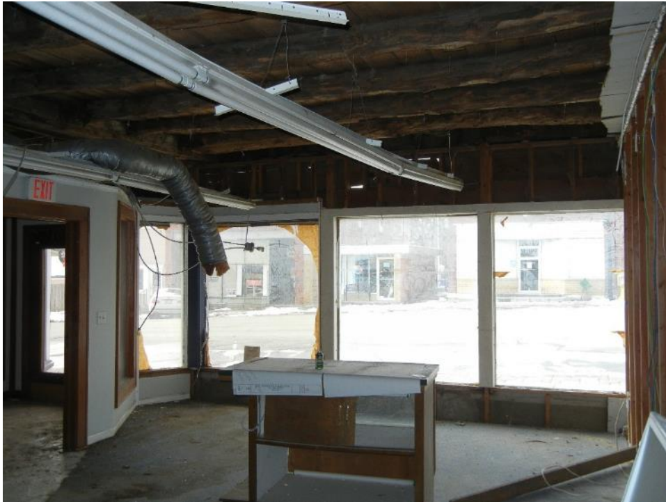
Photo 16: First floor display windows, North section
