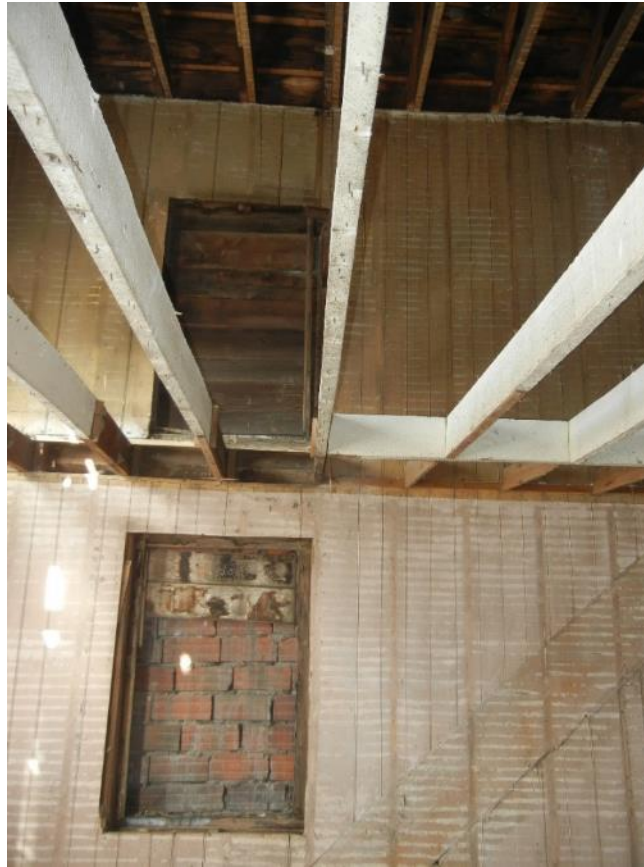
Photo 38: Second floor, north section, exterior openings (covered) and wall finish
