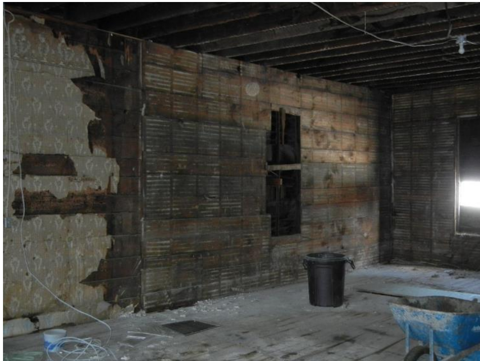
Photo 55: Second floor, south section, north wall (former exterior)
