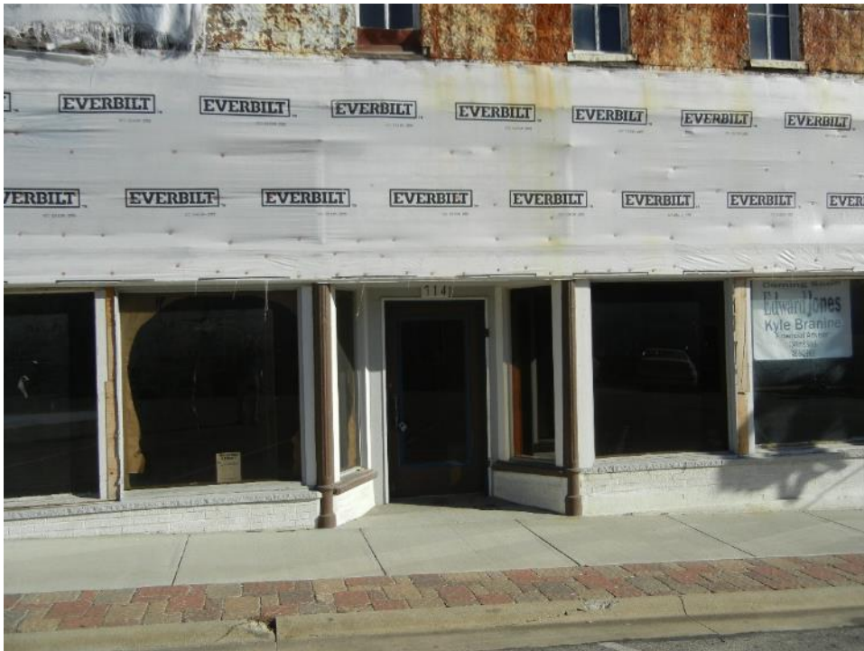
Photo 4: Detail of storefront, central entrance
