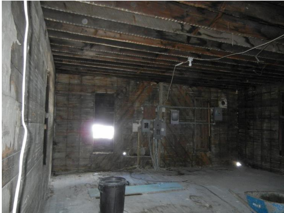
Photo 54: Second floor, south section, rear wall and ceiling joists
