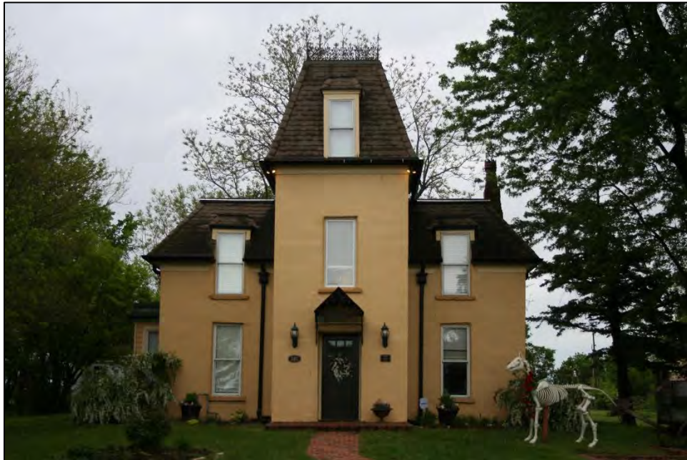
Figure 1. John Brender Residence, Eudora, Douglas County 2019 – North Elevation
