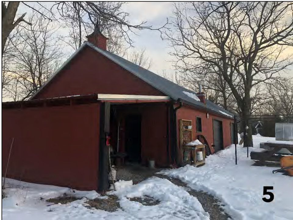
Figure 6. John Brender Carriage House looking southeast – taken by Nolan Jones February 21, 2019
