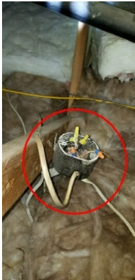
Open electrical junction box in attic
