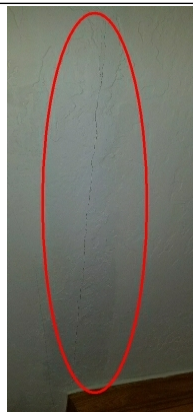
Typical cracking at ceiling
