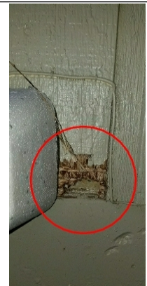
Small damaged area of siding on south side of home
