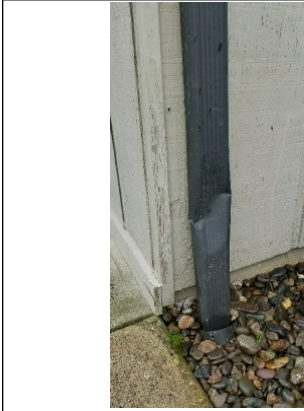
Damaged downspout at NW corner of the home
