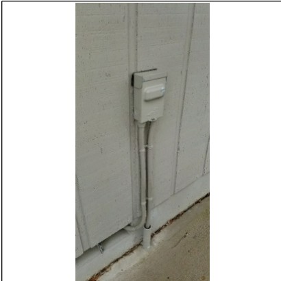
Hot tub power supply and shut-off
