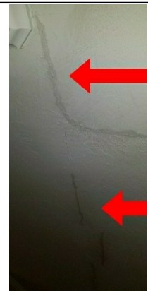
Typical cracking in ceiling
