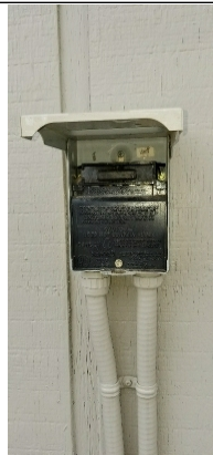
Hot tub power supply and shut-off
