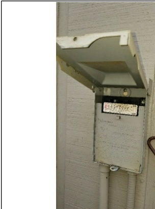
AC unit shut-off
