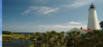
St. Marks Lighthouse
