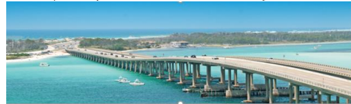
Hathaway Bridge, Panama City to Panama City Beach
