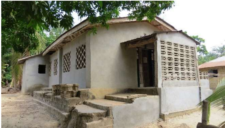
2016 Church Roof project
