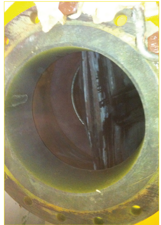
Shown here is the rubber valve inside the metal housing, viewed from the discharge end of the valve.
