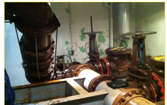
Shown here is the extensive bracing (light gray beams and saddles) connecting the piping to the wall that had been installed after a catastrophic water hammer event had occurred 10 years or so prior to the new valve installation.
