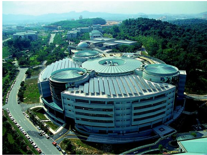
362kWp Off-Grid @ TPM 2001
