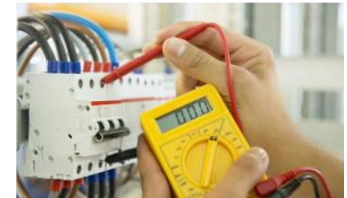
Solar Electronic Protection Switch Inspection
