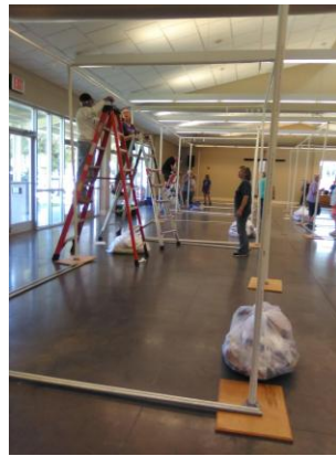
Hanging Rods & Beams for Future Bays
