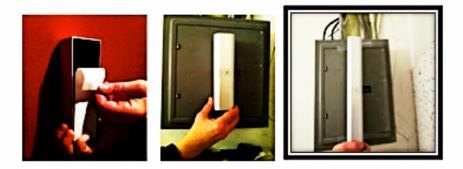
Before letting go of the transformer make sure it is attached strongly to the circuit breaker box door
