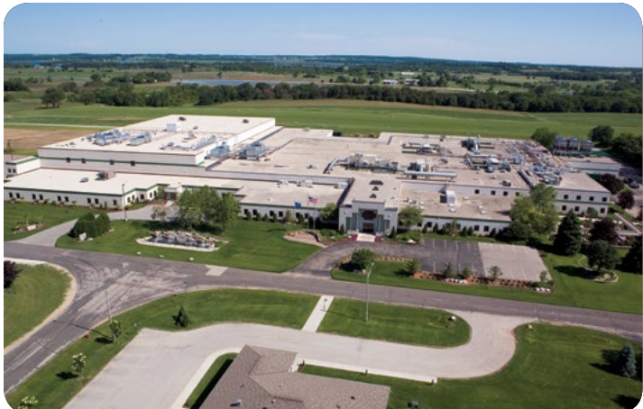
The Standard Process corporate headquarters in Palmyra, Wisconsin, located just down the road from our certified organic farm. This 287,000-square-foot building includes the manufacturing facility and houses the company's 370 employees.
