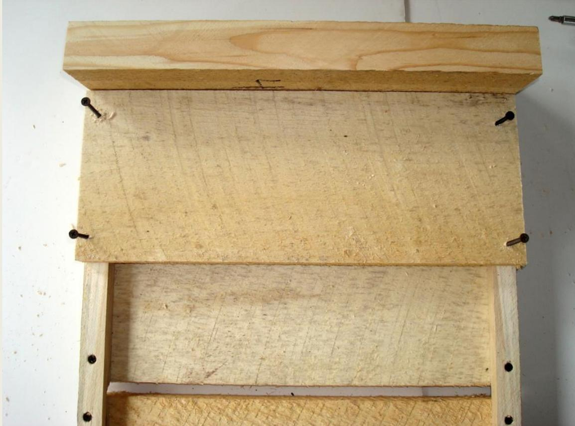
**Attach the first interior baffle with 2" drywall screws.**
