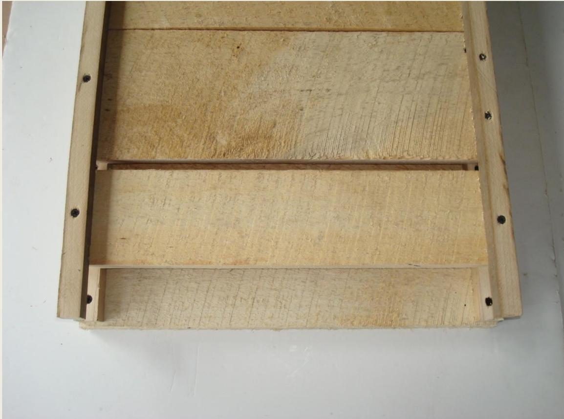
**Attach the 2<sup>nd</sup> row of  $\frac{3}{4}$ " spacers with 2" drywall screws.**
