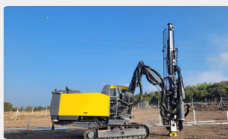
Mobile equipment (excavators and drilling rigs)
