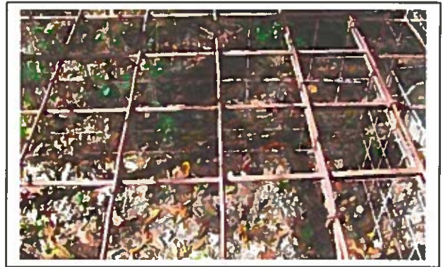
Rusted/pitted wire upper panel
