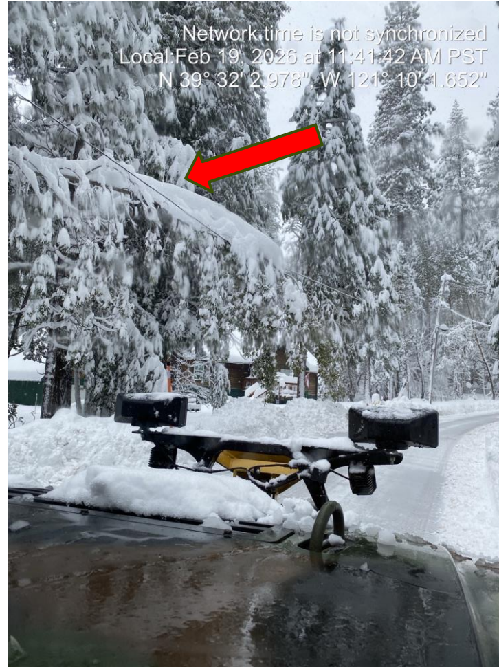
Branches leaning over power lines
