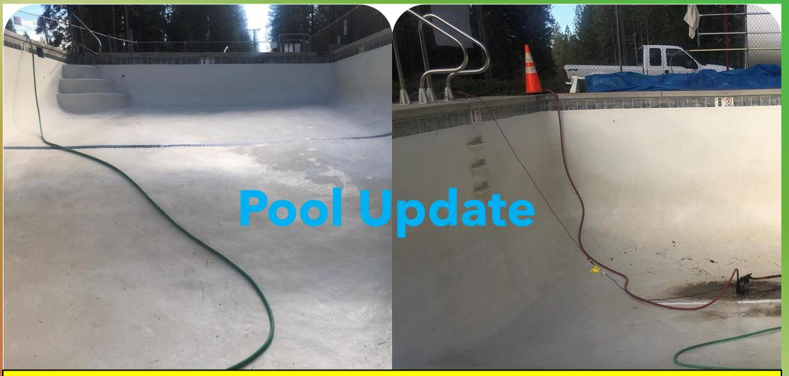
The pool was drained, cleaned, new grates put in and refilled. Water was pumped from the pool into the water tender and replaced from the tender, thus saving precious water–10,000 gallons (estimated).
