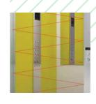
PHOTOELECTRIC CURTAIN Avoids the risk of the doors hitting, allowing a safer use of the lift.
